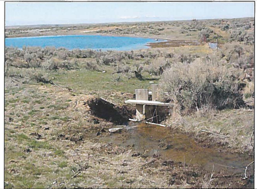
3-13-2014 photograph looking southwest past the washed out diversion structure on the 4-Mile Ditch to the full CDN Upper Ryegrass reservoir in the background. Washout points to higher earlier flows.
