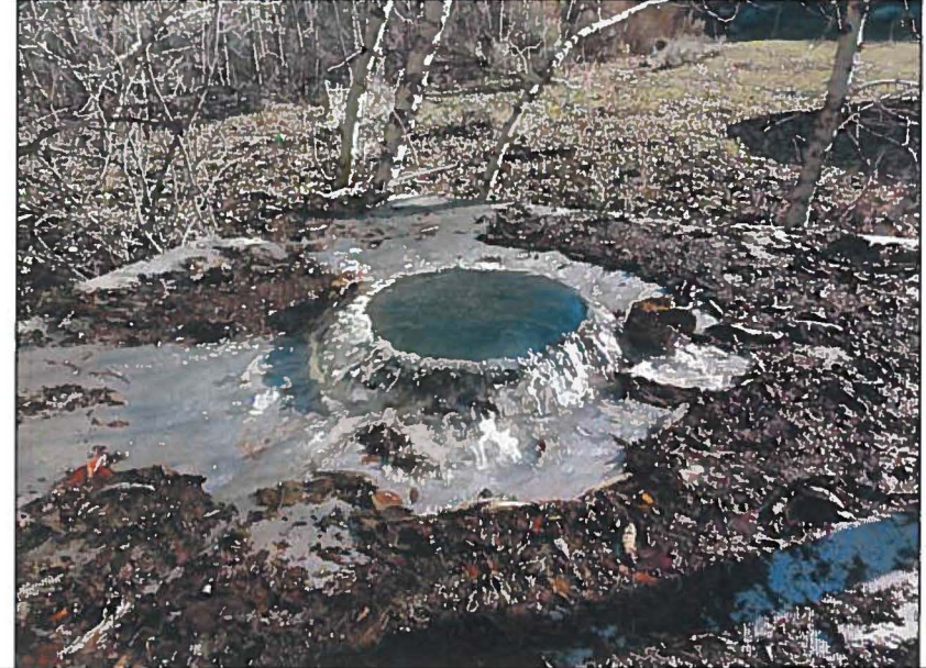
3-13-2014 Cold Springs Creek water entering the CDN bubbler and flowing out on to a trash screen which separates leaves, debris, and the many small fish seen stranded on the screen.
