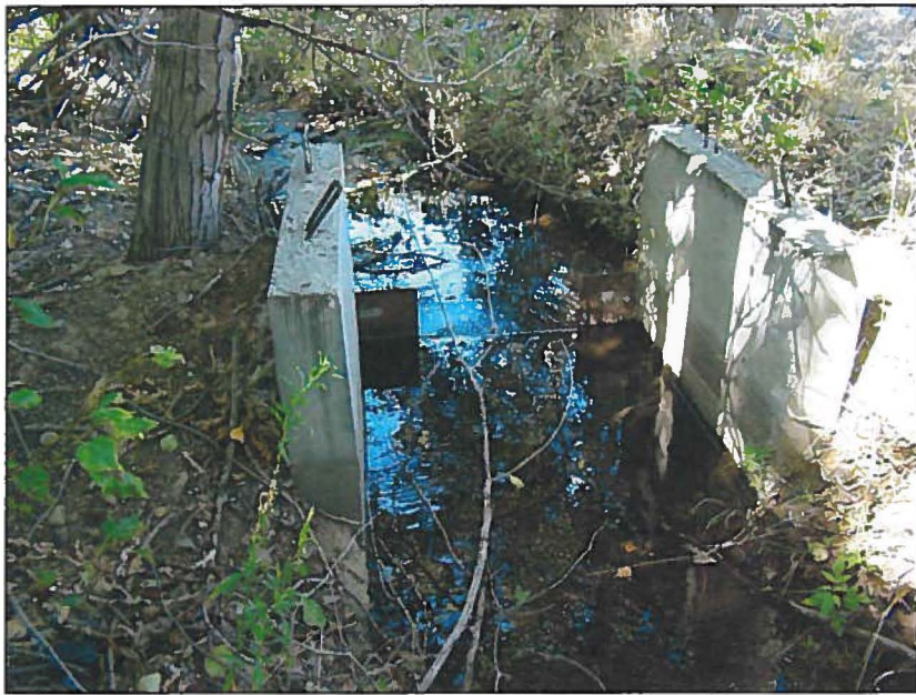
7-22-2013 photograph of the measurement weir for the Elk Pen Ditch just below the CDN's Upper Main Cold Springs Creek Diversion with only a few tens of gallons per minute flowing over the weir plate.
