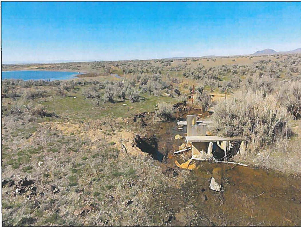
3-13-2014 photograph looking southwest past the washed out diversion structure on the 4-Mile Ditch to the CDN Upper Ryegrass reservoir in the background. Washout points to higher earlier flows.
