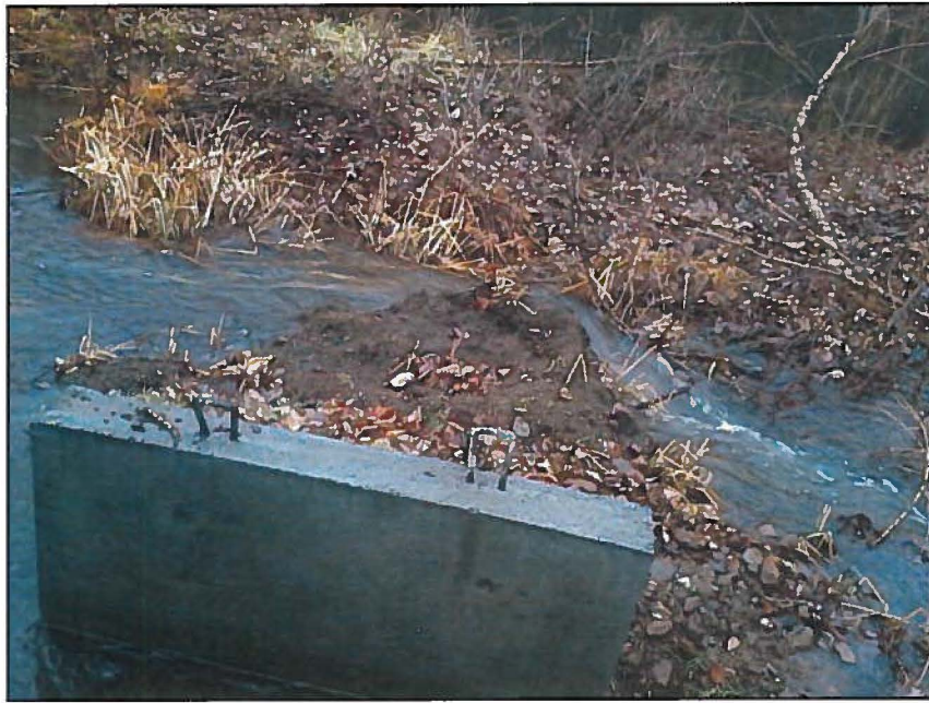
2-14-2014 Photograph by Kelly Riggs and Rich Neal during their site visit to the Casa Del Norte Ranch one day prior to the start of the irrigation season showing a washed out Elk Pen/Four-Mile Ditch Weir.
