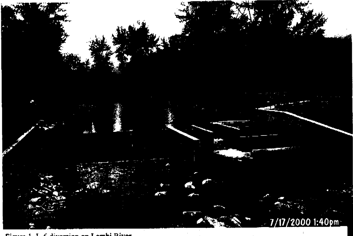
Figure 1. L-6 diversion on Lemhi River. USGS Gauging Station 13305310, Lemhi River Below L-5 Diversion Near Lemhi reading 14 cfs.
