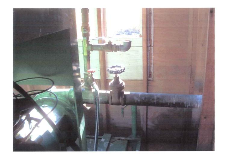
Gate Valve on discharge Pipe - Point of lockable Control
