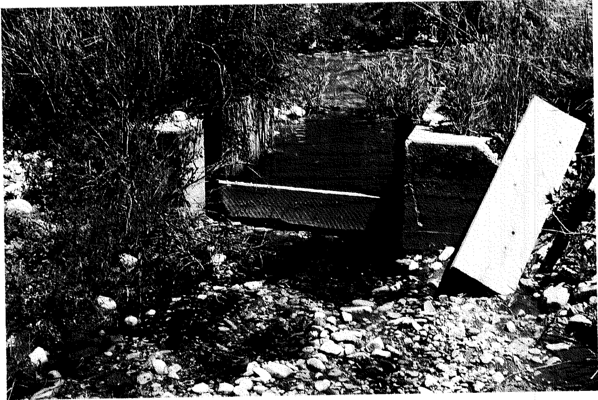
This is the Hoskins headgate with approximately 0.1 cfs coming under the board and through the rocks.
