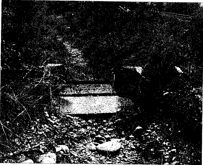
25: LARRY KEMPTON SOUTH WEIR
