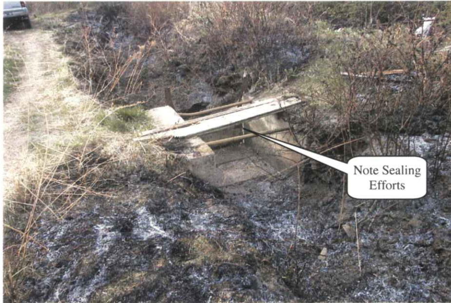
ABOVE & BELOW: Views of measurement point on the Lower West Ditch. Efforts had been made to repair this weir. During the visit, some water was turned down this ditch and it appeared that this weir was functional with very minimal leakage. Note efforts made to seal edges of weir to prevent leakage around the weir.
