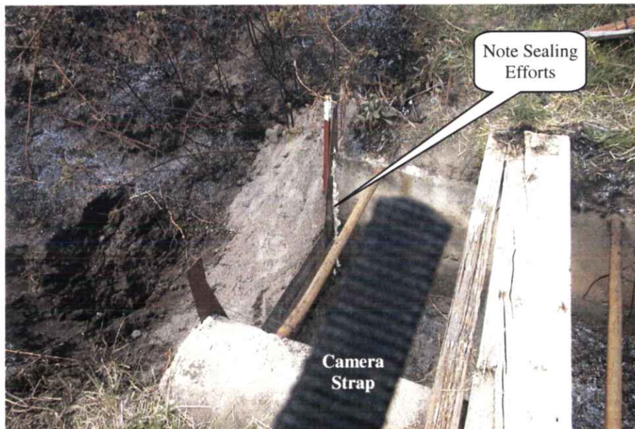
ABOVE & BELOW: Views of measurement point on the Lower West Ditch. Efforts had been made to repair this weir. During the visit, some water was turned down this ditch and it appeared that this weir was functional with very minimal leakage. Note efforts made to seal edges of weir to prevent leakage around the weir.
