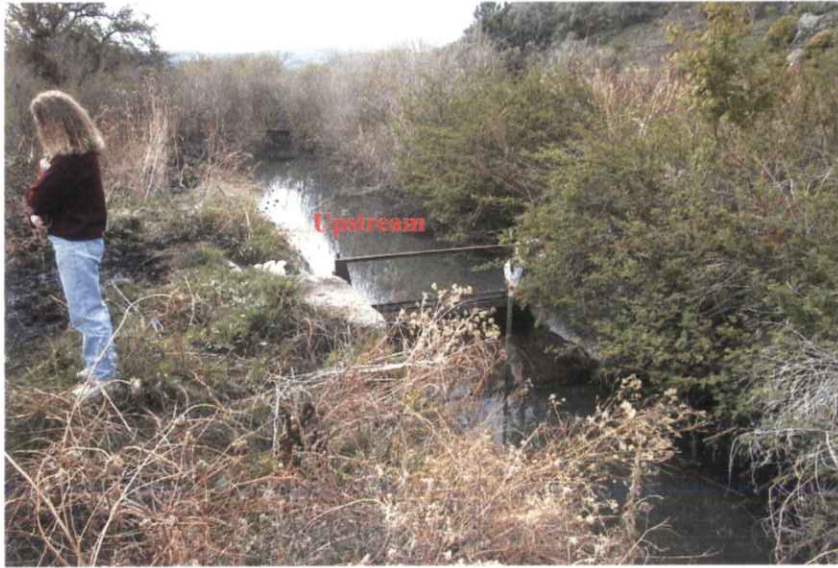
ABOVE & BELOW: Views of measurement point on the Upper West Ditch. Rather recently, efforts had been made to repair this weir. Efforts to repair this weir consisted of attempting to seal the upstream side with a plastic tarp and sand bags (photo below). Note that water adjusted in ditch so that no water is flowing over this weir. Water downstream of view can be contributed to continued leakage &/or water spilled over weir before water was adjusted in ditch or before efforts were made to repair the weir.
