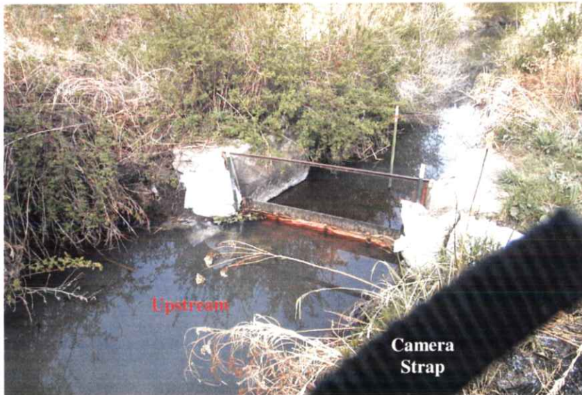
ABOVE & BELOW: Views of measurement point on the Upper West Ditch. Rather recently, efforts had been made to repair this weir. Efforts to repair this weir consisted of attempting to seal the upstream side with a plastic tarp and sand bags (photo below). Note that water adjusted in ditch so that no water is flowing over this weir. Water downstream of view can be contributed to continued leakage &/or water spilled over weir before water was adjusted in ditch or before efforts were made to repair the weir.
