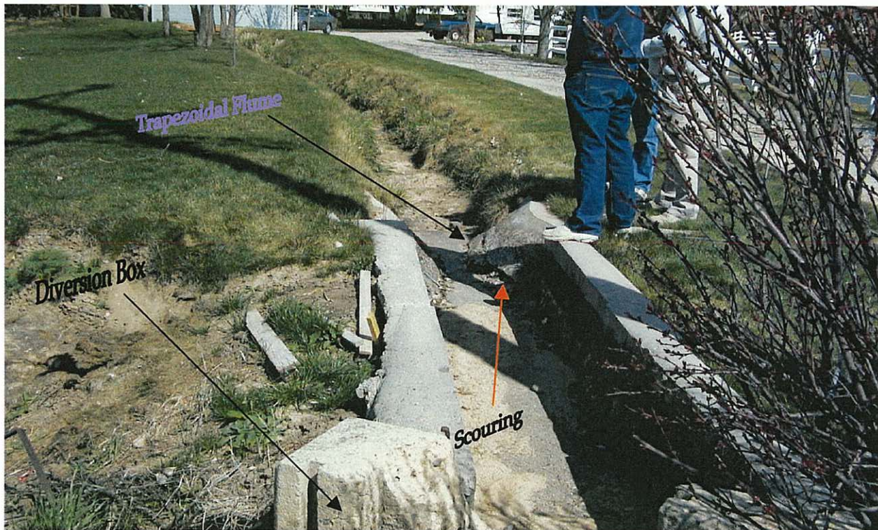
Photo #2: Hally-Scott Ditch from the diversion box.
