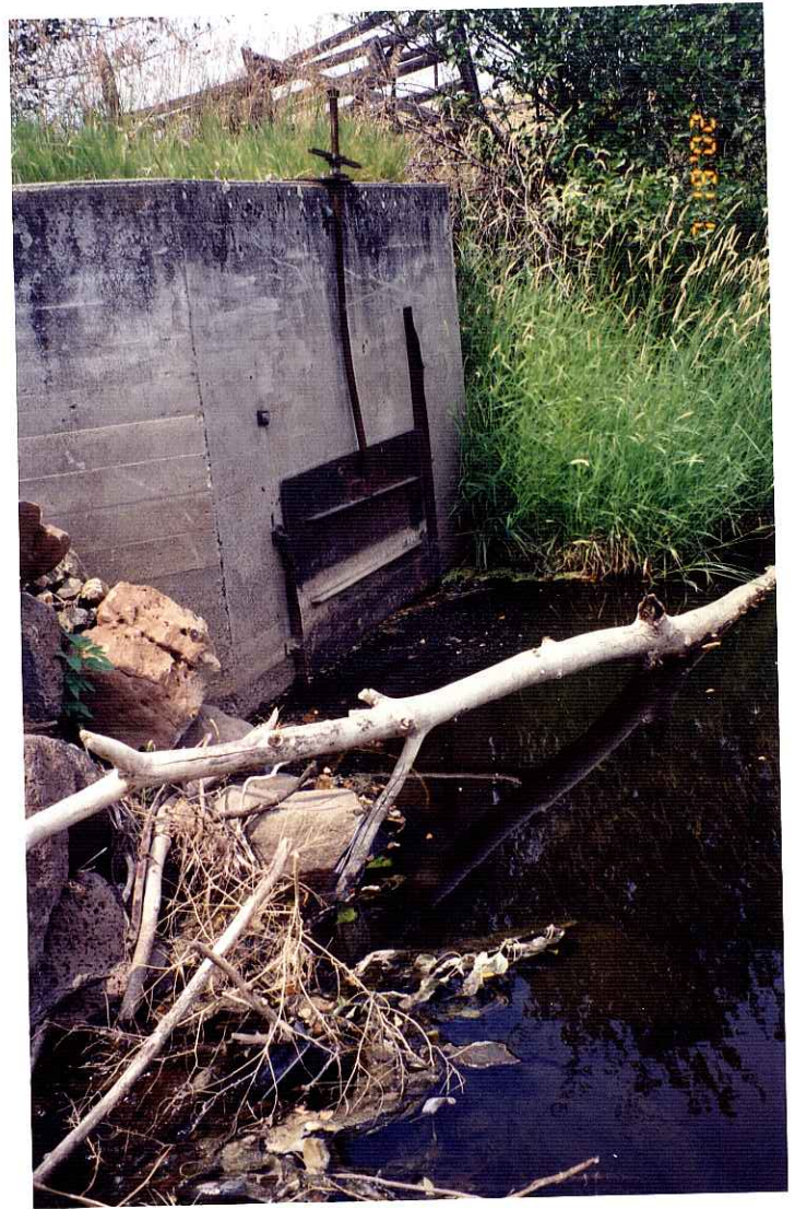
Wilkinson Ditch Headgate
