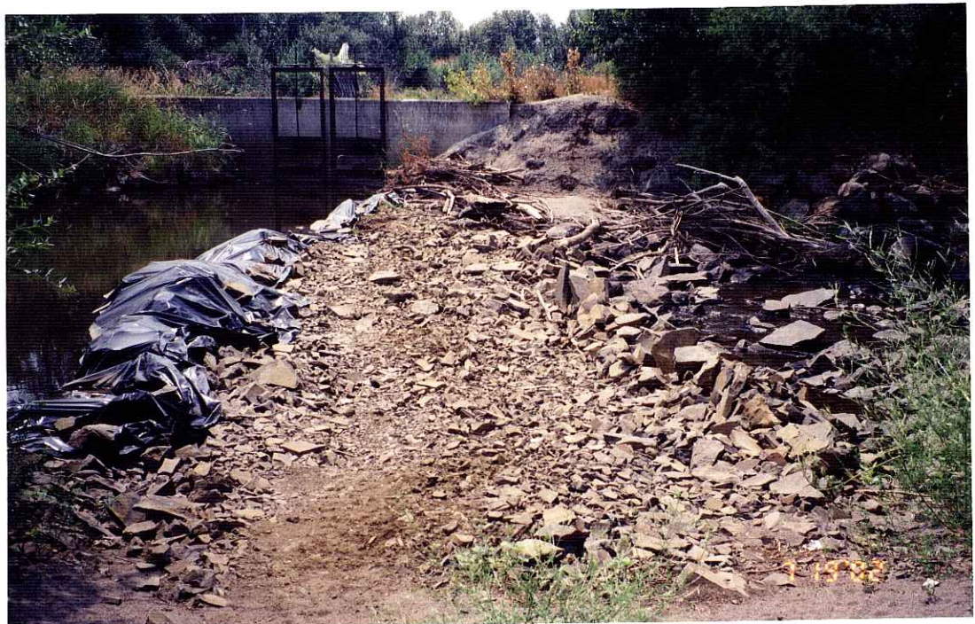
Schwenkfelder Ditch Headgate
