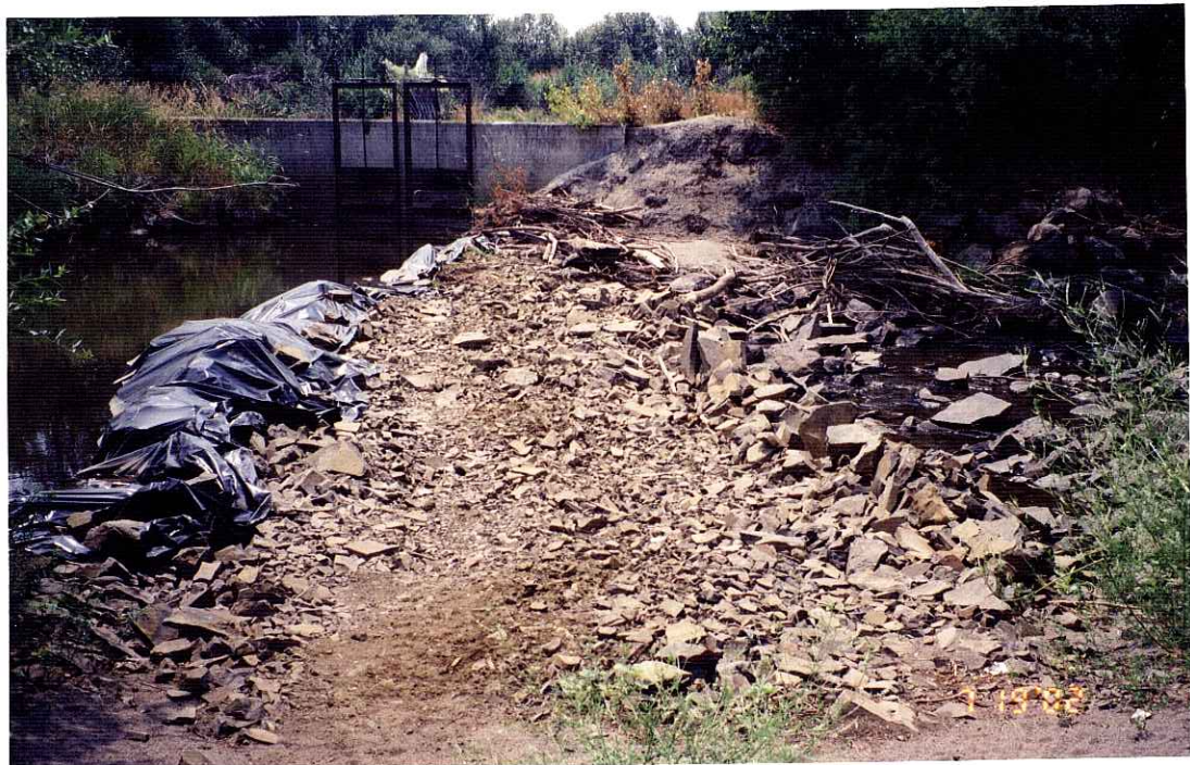
Schwenkfelder Ditch Headgate
