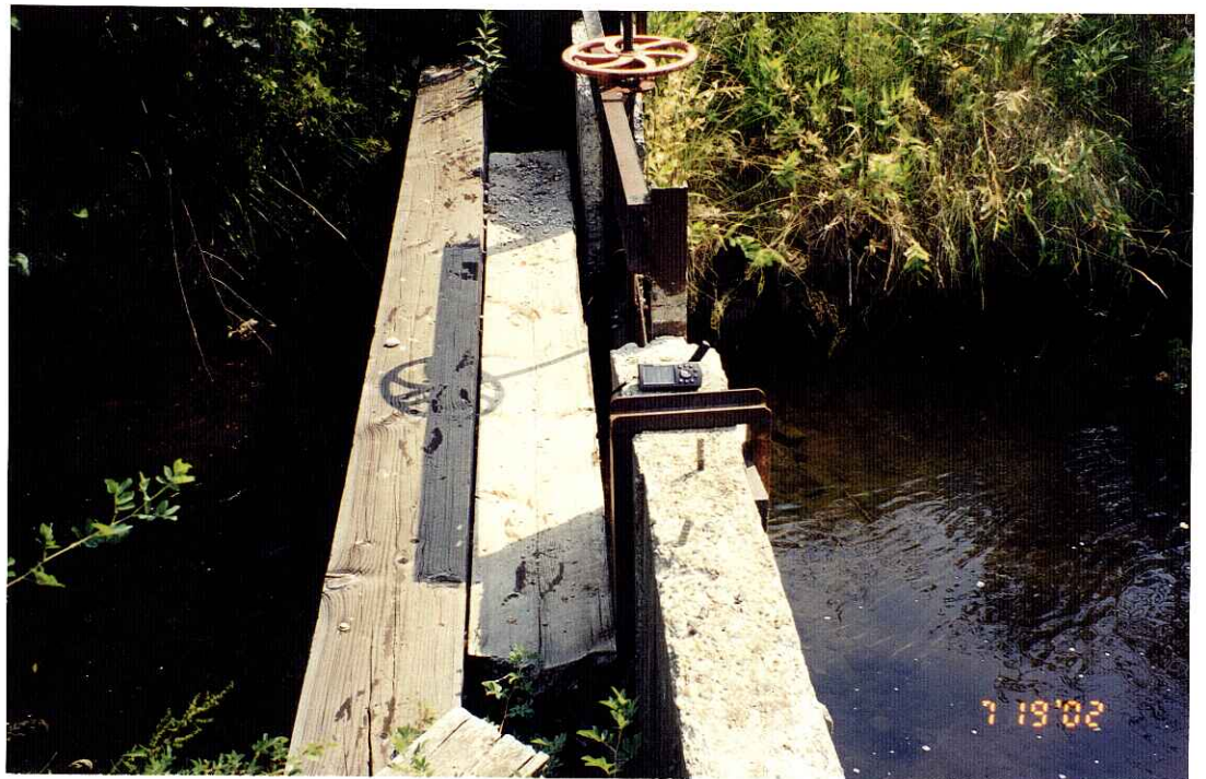
American / Lindsey Ditch Headgate
