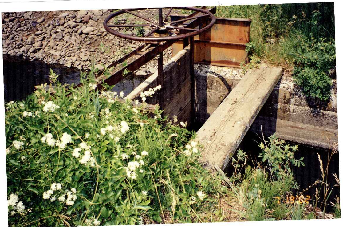
Greys Creek Ditch Headgate
