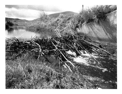
**Little Camas Creek:** Eight measurements were taken at Little Camas Creek, done at 3 points/culverts that pass under Highway 20. Culverts designated as **LC1**, **LC2**, and **LC3**. The rating curve developed was an average of the three culverts. As with Cat Creek, beaver construction obstructed/altered flows between measurements.
