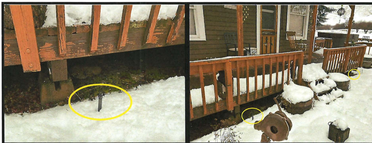
Photo 12a & b- Fan sprinklers found in bedding and at shrubs around the house.
