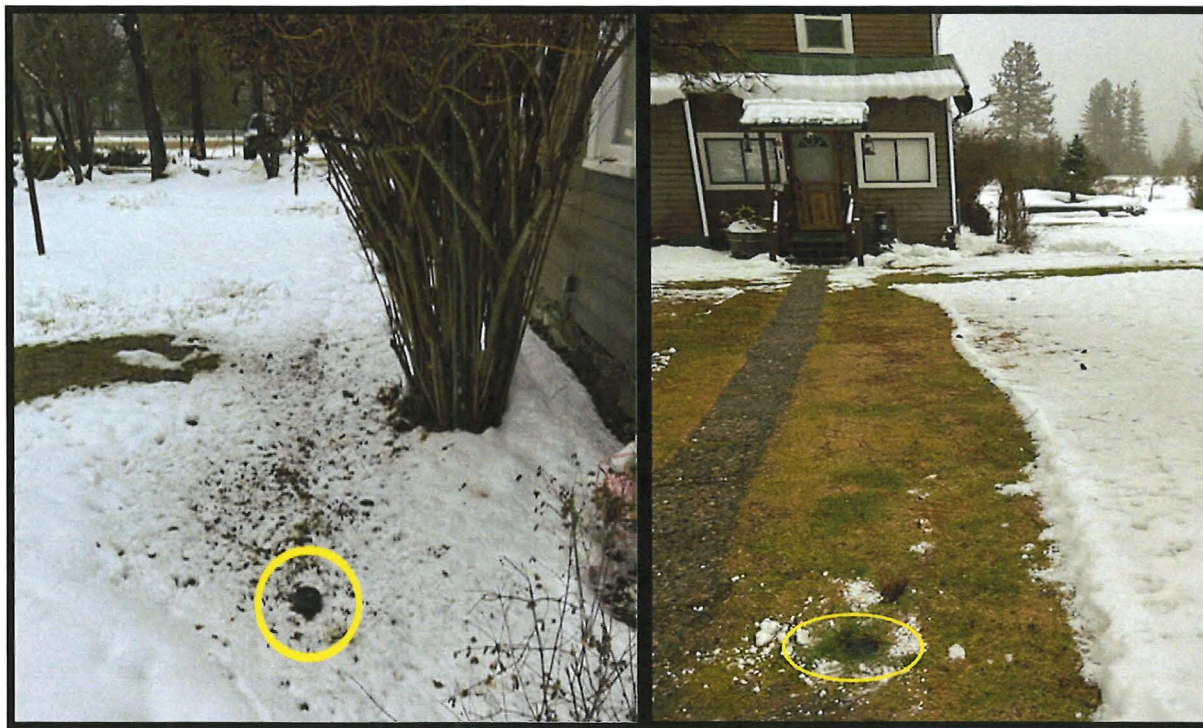
Photo 11a &b- Rain Bird rotary sprinklers within the POU.
