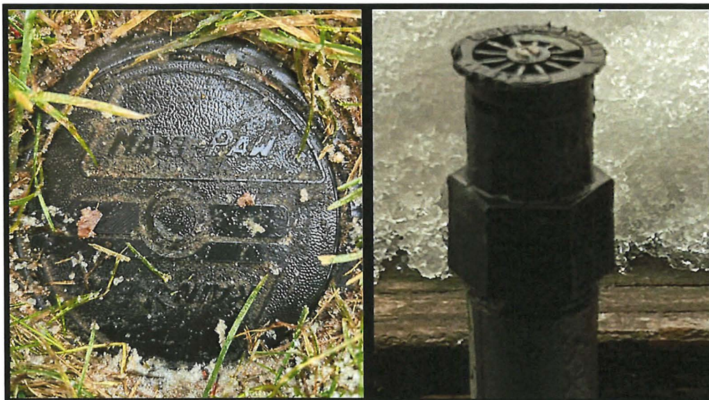
Photo 10a-(left) Rain bird Maxi-Paw sprinkler heads found in 8 zones of the POU. Photo 10b-(right) Fan sprinklers found in landscape beds and near shrubs around the house.
