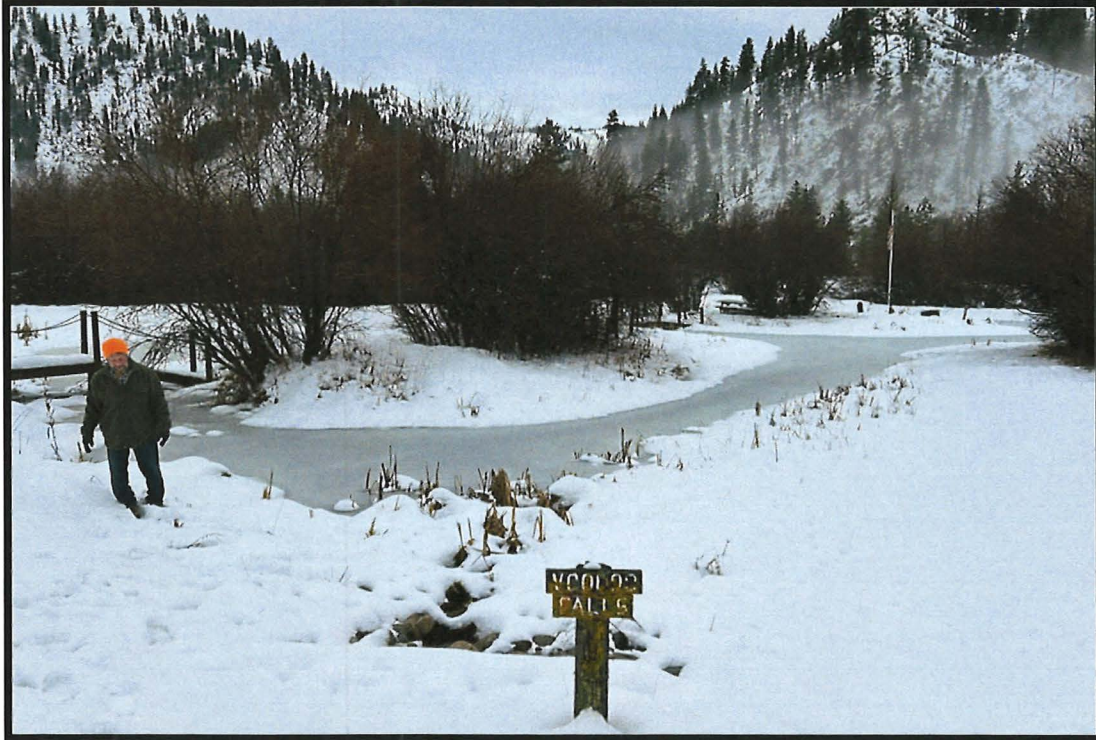
Photo 3- North of the pond facing south. The discharge of the 6" PVC pipe into the pond just past "Voodoo Falls" sign.
