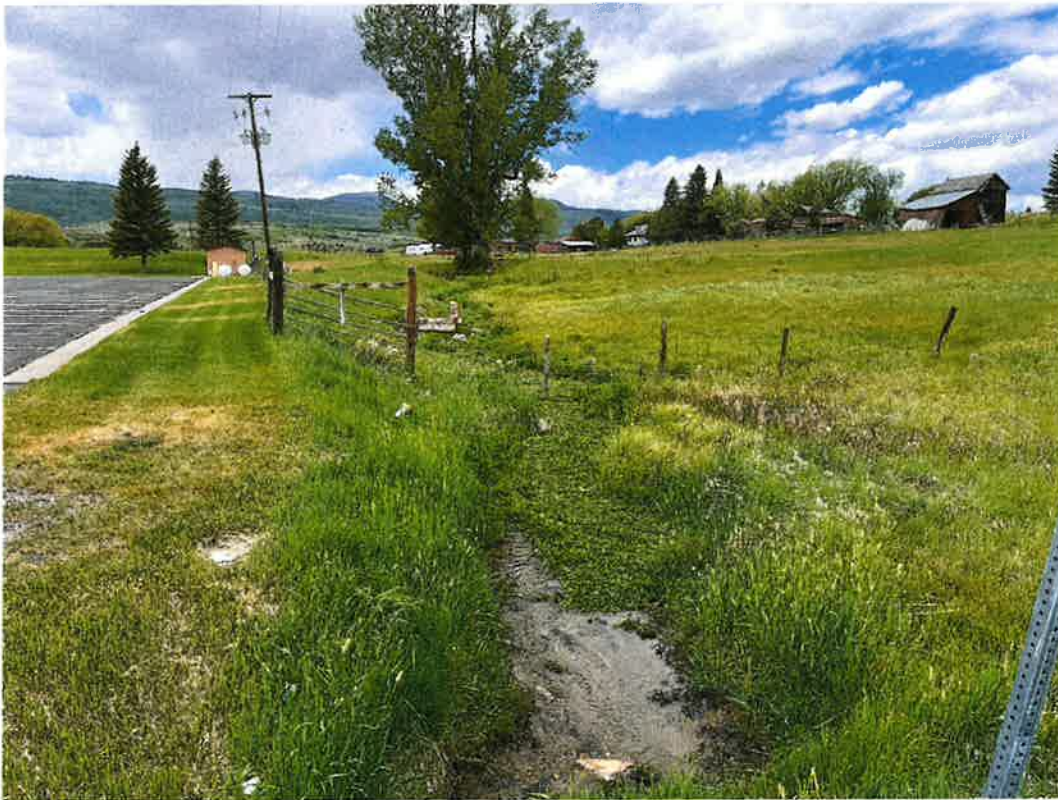
Spring flowing from the base of the tree, picture downstream looking up.
