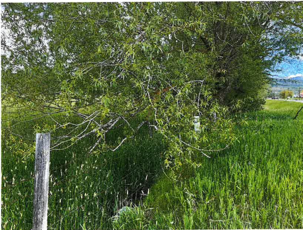
Western most culvert under the highway reaching the southern POU.
