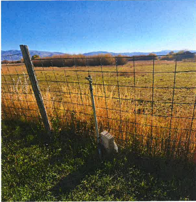
Figure 17: South riser with affixed impact sprinkler behind the home at the Bergs residence.
