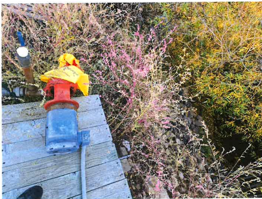
Figure 2: Irrigation pump assembly platform affixed atop creek bench.
