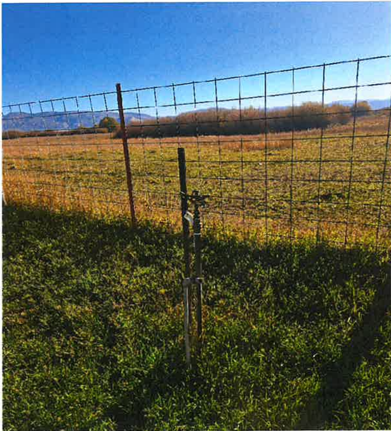
Figure 18: North riser with affixed impact sprinkler behind the home at the Bergs residence.
