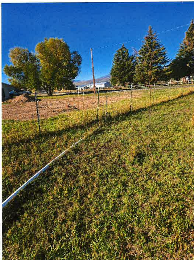
Figure 16: The above ground conveyance line attaches to a riser with an affixed impact sprinkler on the south side of the residence.
