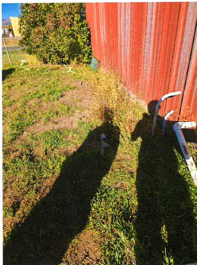
Figure 20: Riser located next to the hay shed in-between the residence and the shed at the Bergs residence.
