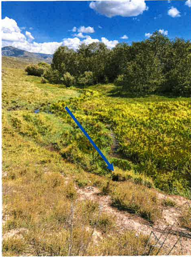
Photo 5: Standing on dam looking upstream.
