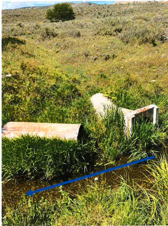
Photo 7: Diversion for north field.
