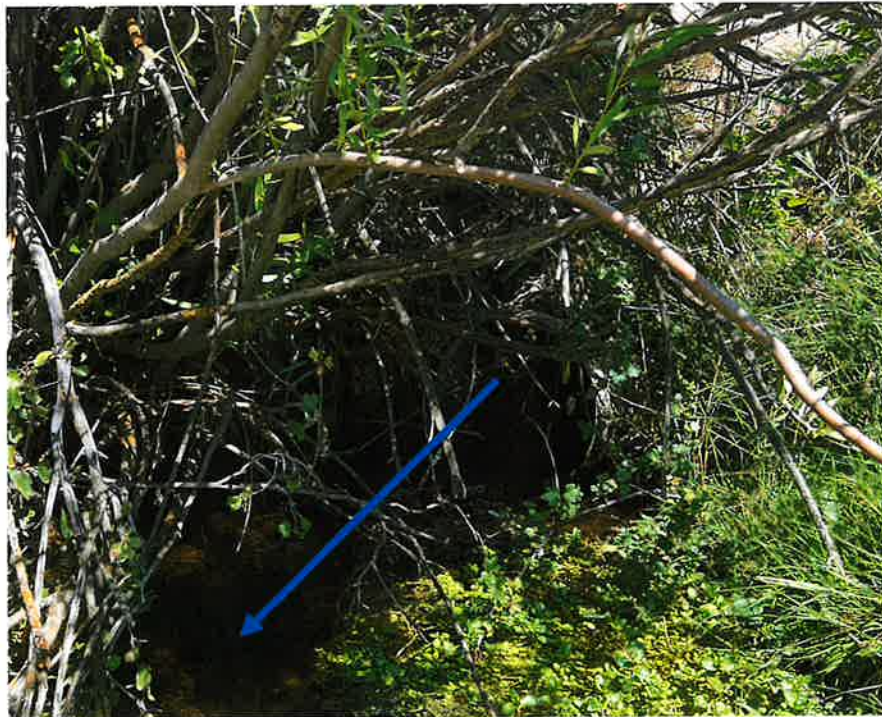
Photo 6: Culvert through bottom of dam.
