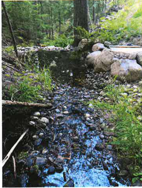
POD: Overview depicting surface water intake area, showing natural creek flow entering the culvert housing where the diversion pump and fish screen are sited.
