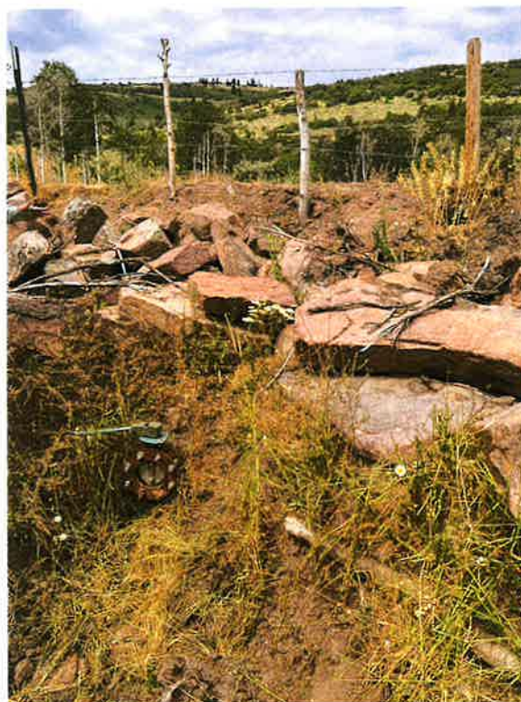
Photo 2: South pond flush valve.
