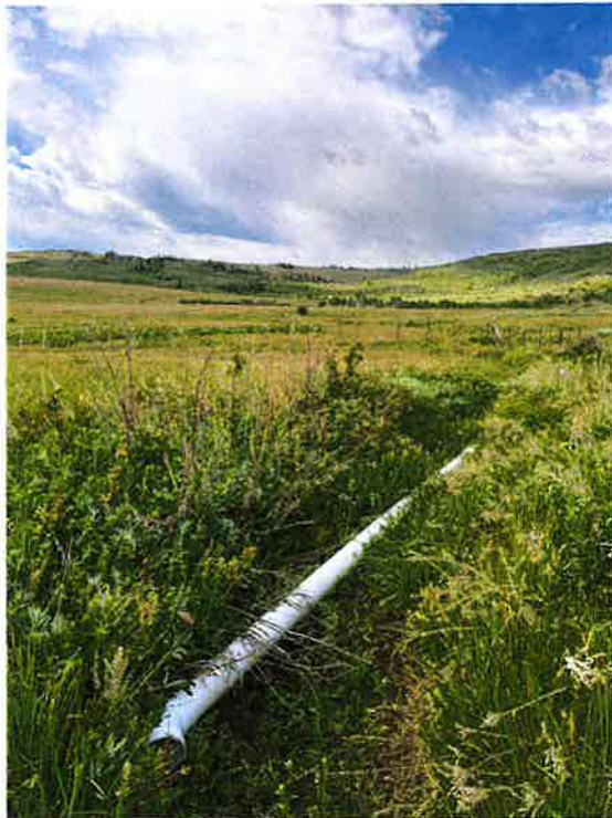
Photo 4: Pipeline from south pond.
