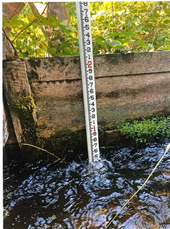
Photo 4: South side of headgate.
