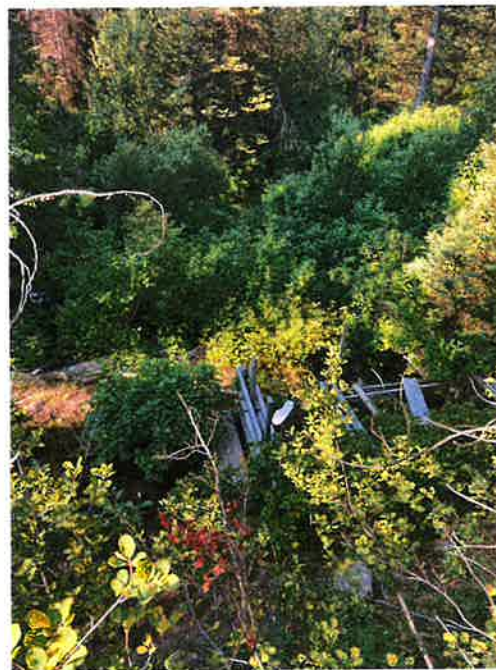
Photo 2: Diversion works from above.
