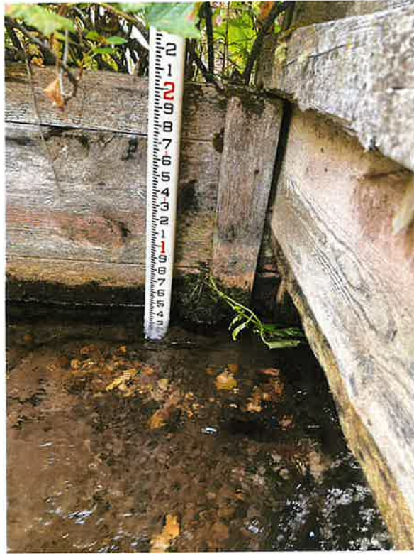
Photo 5: North side of headgate.
