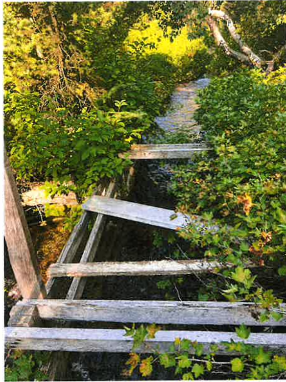
Photo 3: Diversion works with Liberty Creek (top) & return flow (left).
