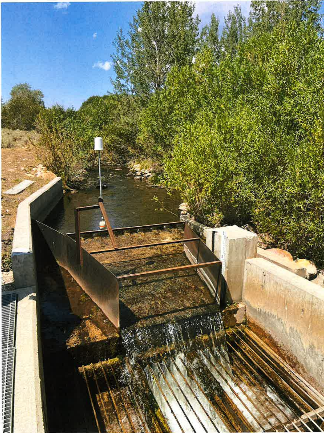
Photo 1: Diversion works looking upstream.
