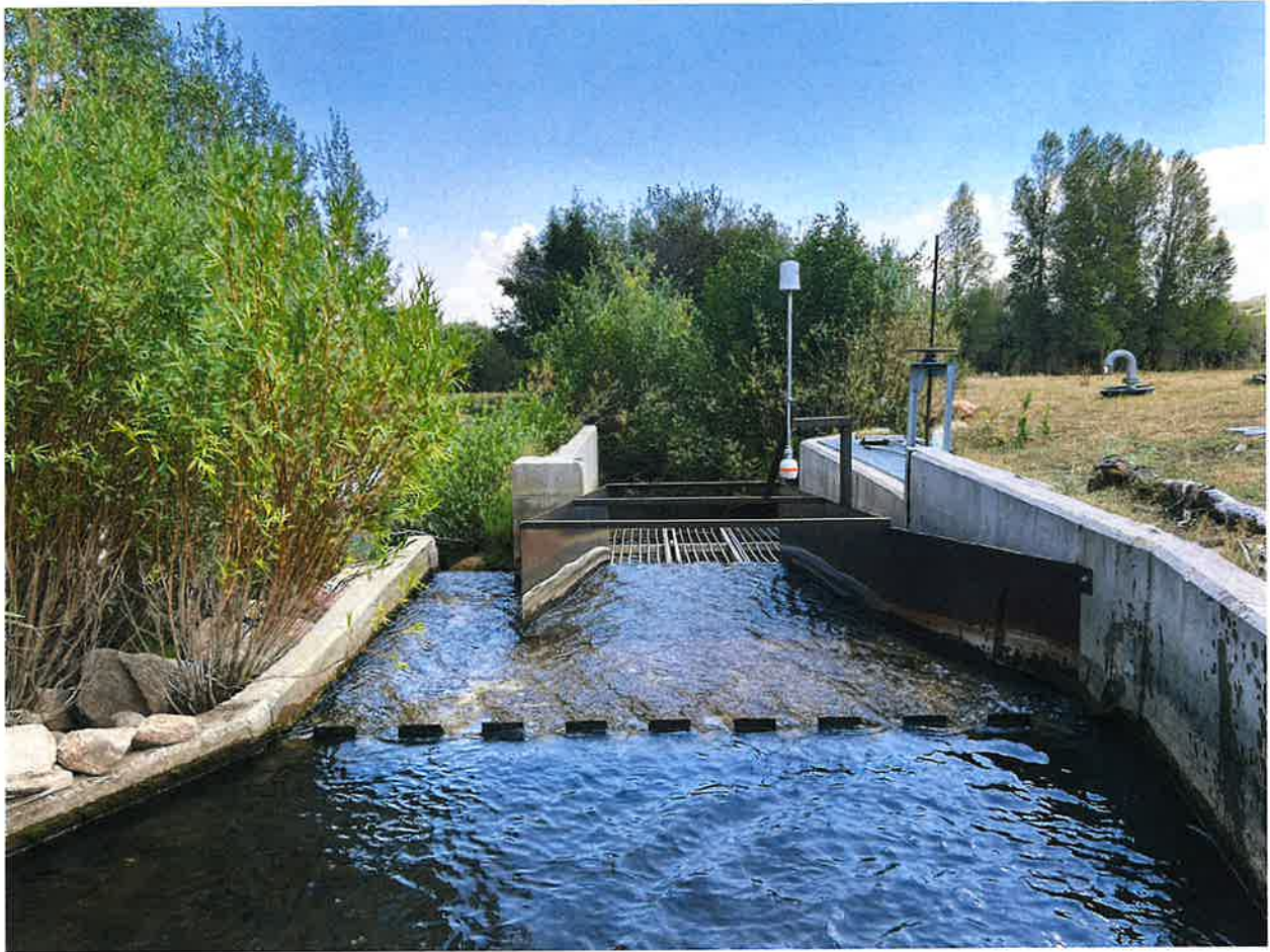
Photo 2: Diversion works looking downstream.
