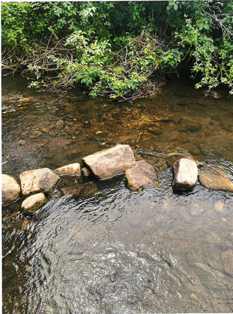
Photo 1: Rock diversion on Mill Creek.
