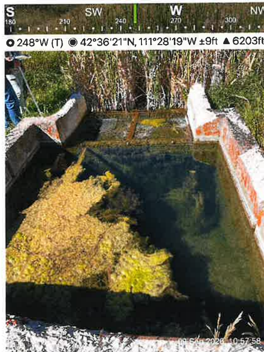
Figure 3: Screen that transfers the water to a pipe. This water is supplied by the headgate in figure 2.
