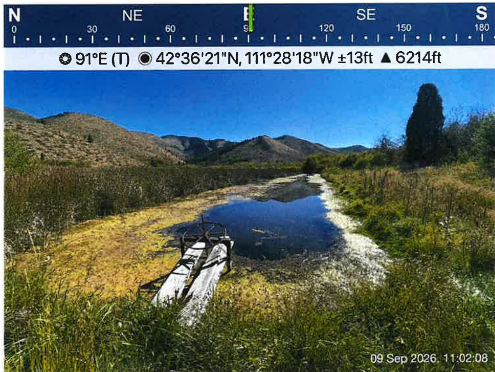
Figure 2: Second headgate that diverts water from the canal to a screen.
