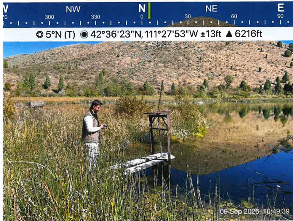
Figure 2: Second headgate that diverts water from the canal to a screen.
