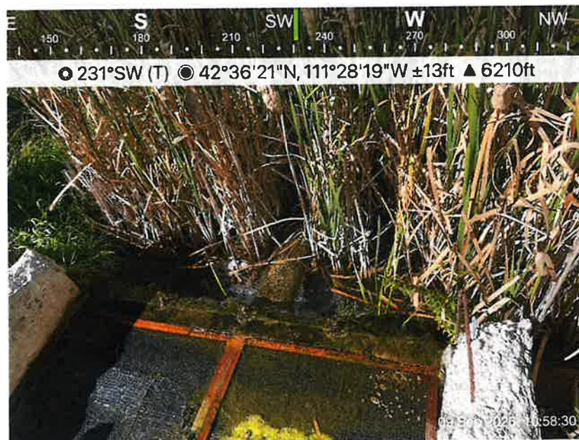
Figure 4: Pipe that takes the water from the screen in Figure 3.
