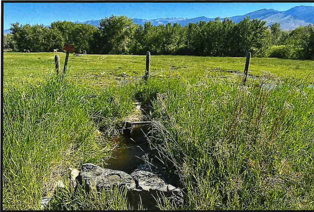
Photo 3- On the north side of the road facing north the channel exiting the weir is mostly symmetrical until it crosses under the fence into the field.
