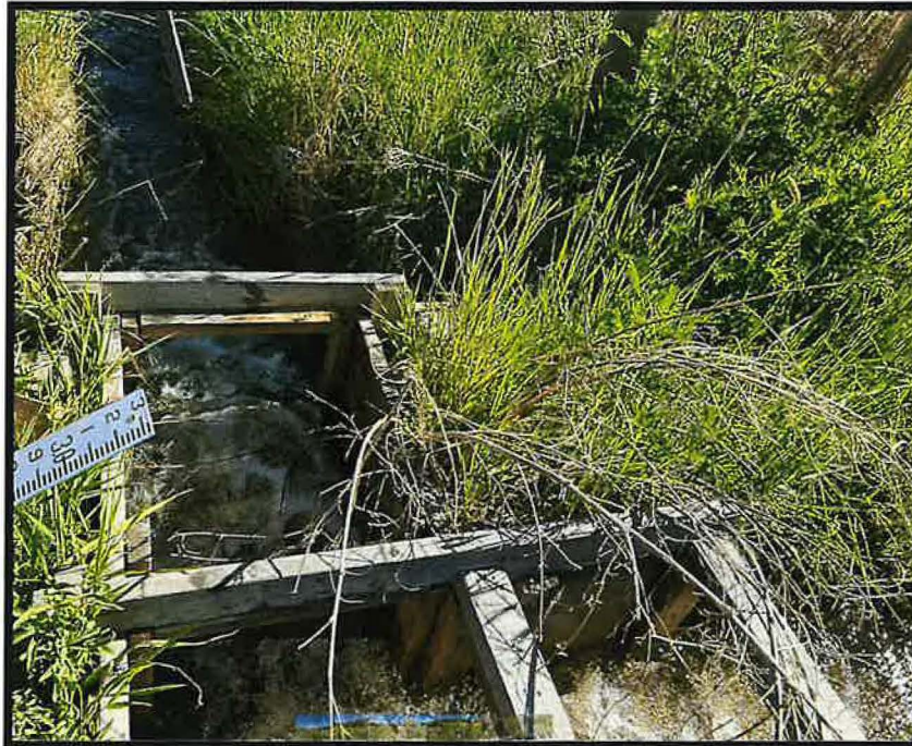
Photo 1- Wooden flat weir facing north. The diversion to the POU runs north and the ditch returning directly to the Lemhi River exits to the east (right of photo).
