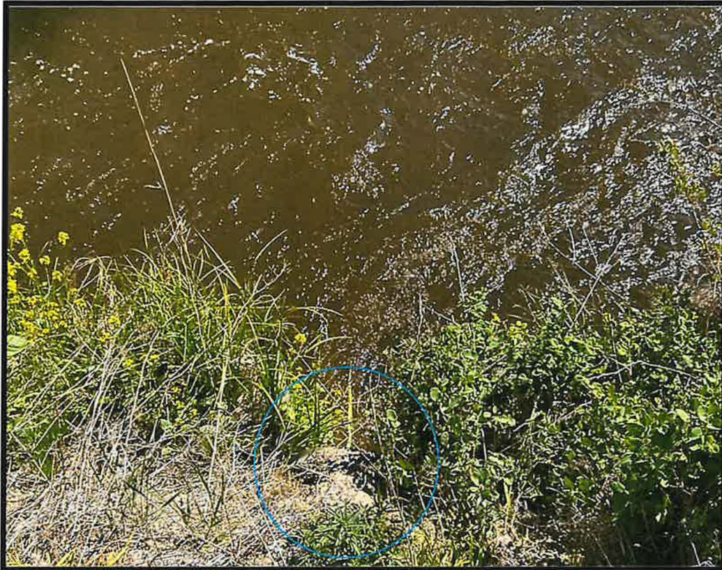
Photo 3- Culvert discharging into the irrigation ditch on the south side of the road. The ditch carries water to lateral irrigation ditches throughout the POU.
