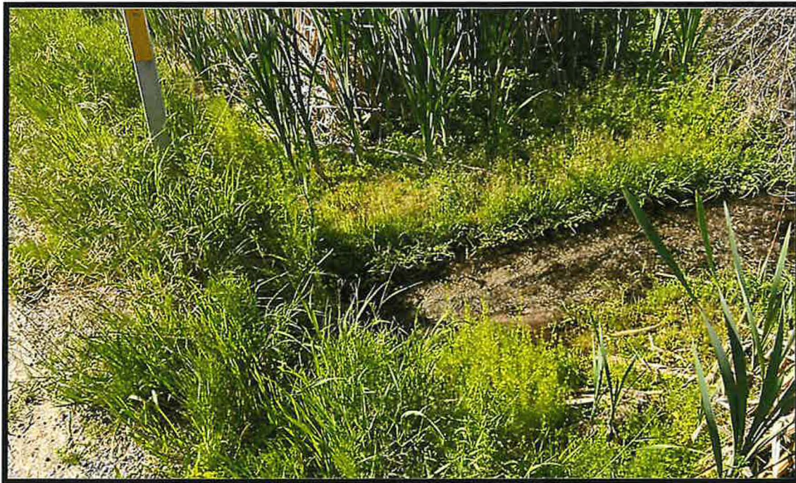
Photo 2- Spring flow entering corrugated steel culvert passing under the road.
