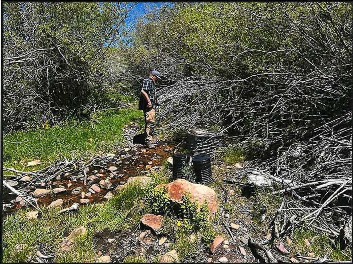
Photo 1- Facing south, standing at the confluence of the spring (source) and McGinty Creek. A metal culvert is used as a shallow spring box with a screened intake submerged to divert water from the spring through a buried downhill to the water trough within the stockwater POU. The black culverts were installed previously for an abandoned system.
