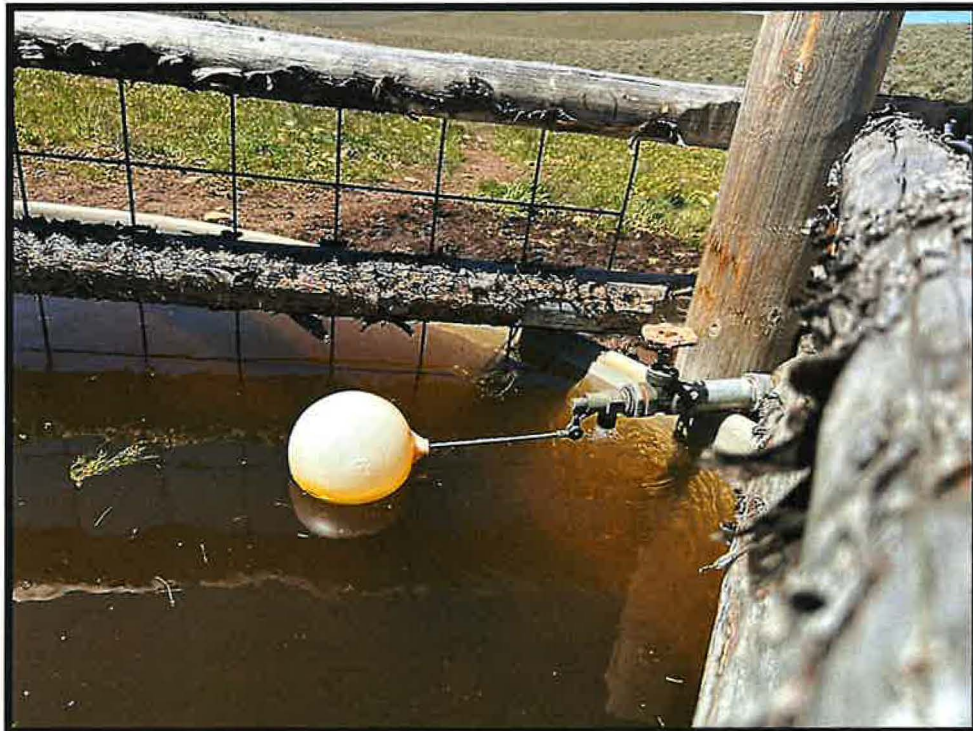
Photo 4- Facing northwest, the float valve mechanism on a 1" valve reduced from the 1 ½ inch steel pipe delivering water from the spring to the southeast. Although there is a drain plug in the tank, at the time of examination the tank was full and could only be drained enough to observe a pipeful flow .
