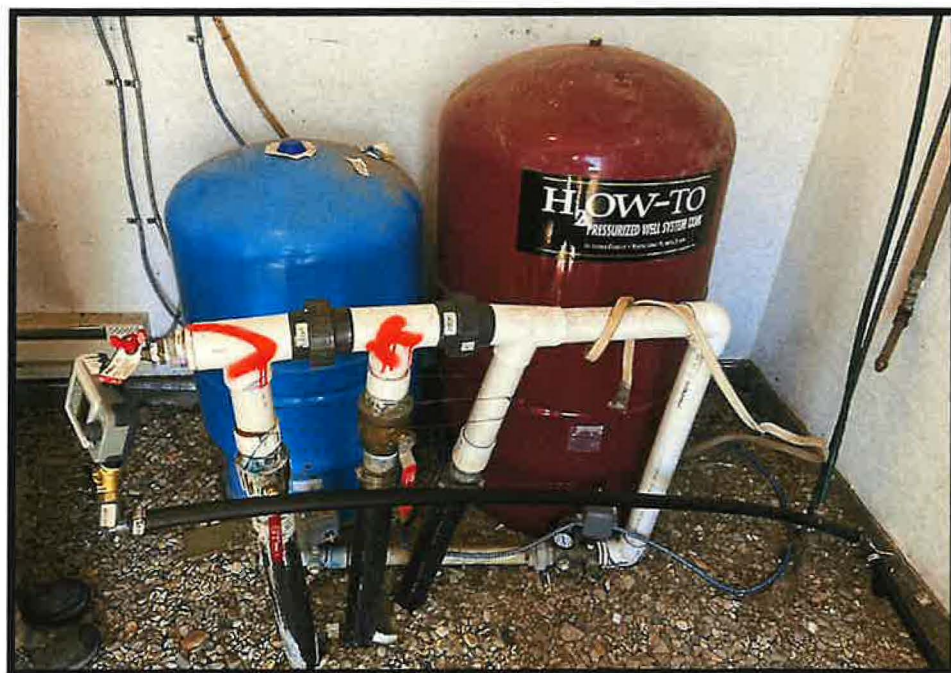
Photo 2- (above) The poly line from the wellhead is the right of the 3 lines between the manifold and the pumphouse floor. The two black lines with hand valves are 2' poly lines delivering water to the hook ups for the trailer park units. Two pressure tanks, one 44-gallon (blue tank) and one 60-gallon (red tank), help maintain pressure when the system is under an increased demand.
