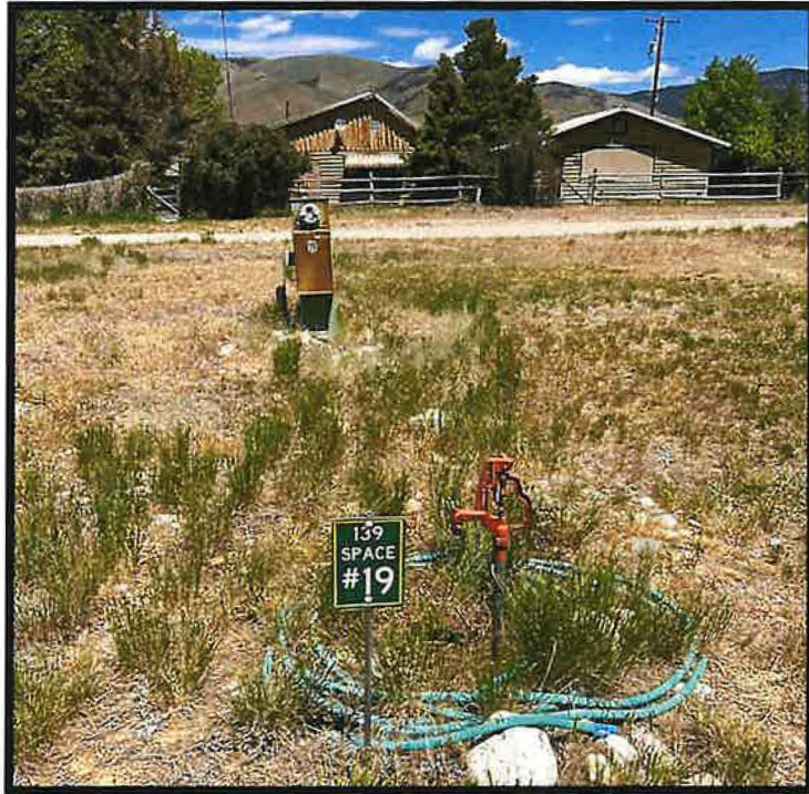
Photo 5-(above) Trailer service near the end of the southeast extent of the POU. The orange frost-free hydrant pictured was used to perform bucket-fill trials. Photo 6- (below) Typical service connections found throughout the trailer park. The blue frost-free hydrant can be seen in the image on the right side of the 4" sewer hookup with blue plug.
