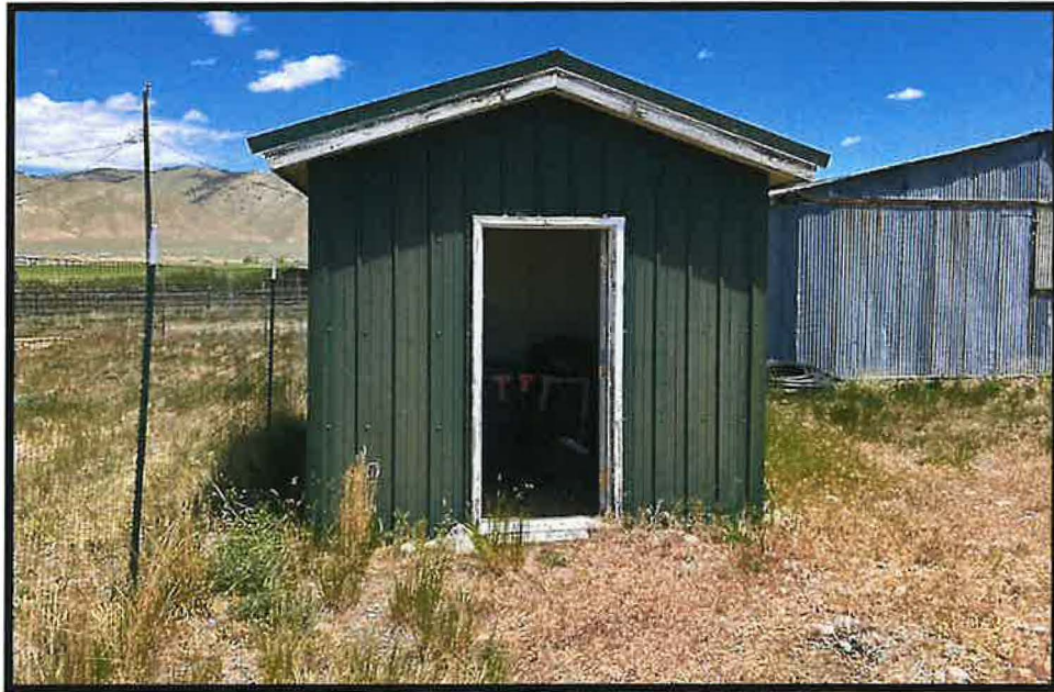
Photo 1- (above) Pumphouse located near the center of the row of trailer units.
