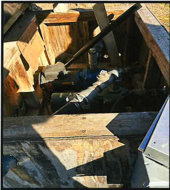
Photo 7 (Left)- The upper pump in the image is for the Irripod system. The lower pump is for neighboring irrigation.
