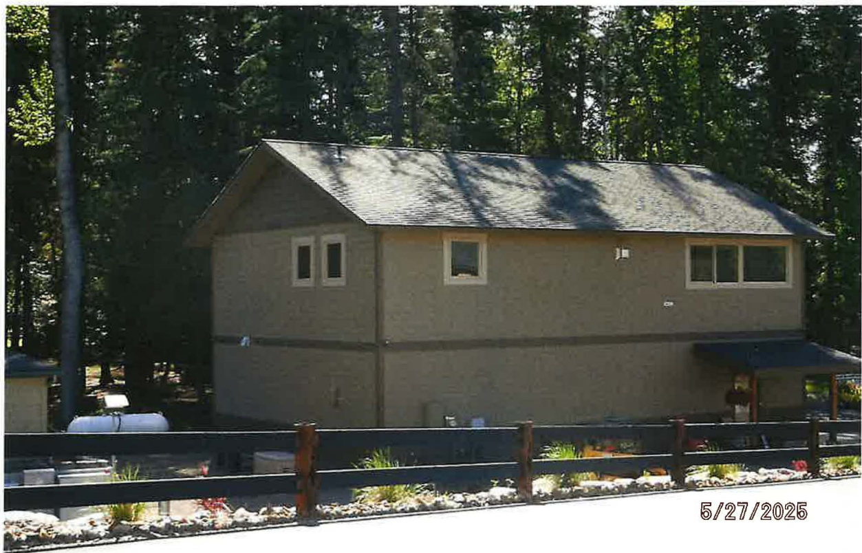
PUMP STATION LOCATED WITHIN THE GRANDVIEW CONDOMINIUMS COMMON AREA CARETAKER RESIDENCE (LOWER LEVEL BACK OF SHOP)
