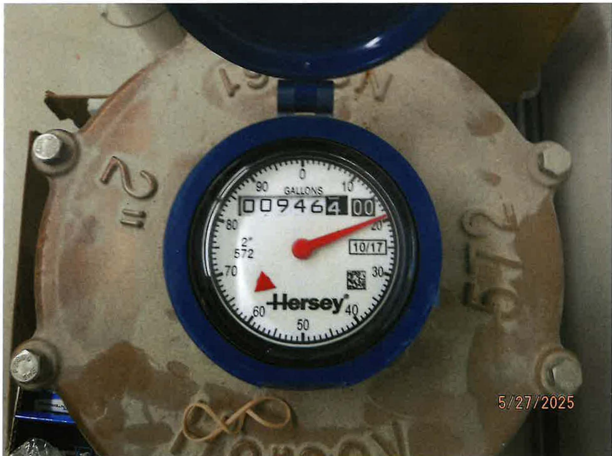
HERSEY FLANGE MOUNTED VELOCITY STYLE FLOWMETER; S/N 18173122; 2-INCH DISCHARGE ORIFICE
