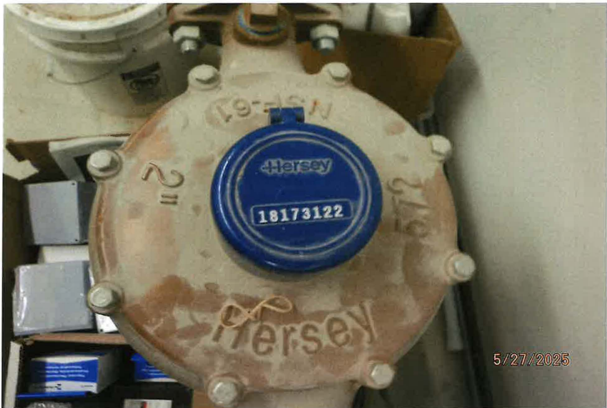
HERSEY FLANGE MOUNTED VELOCITY STYLE FLOWMETER; S/N 18173122; 2-INCH DISCHARGE ORIFICE
