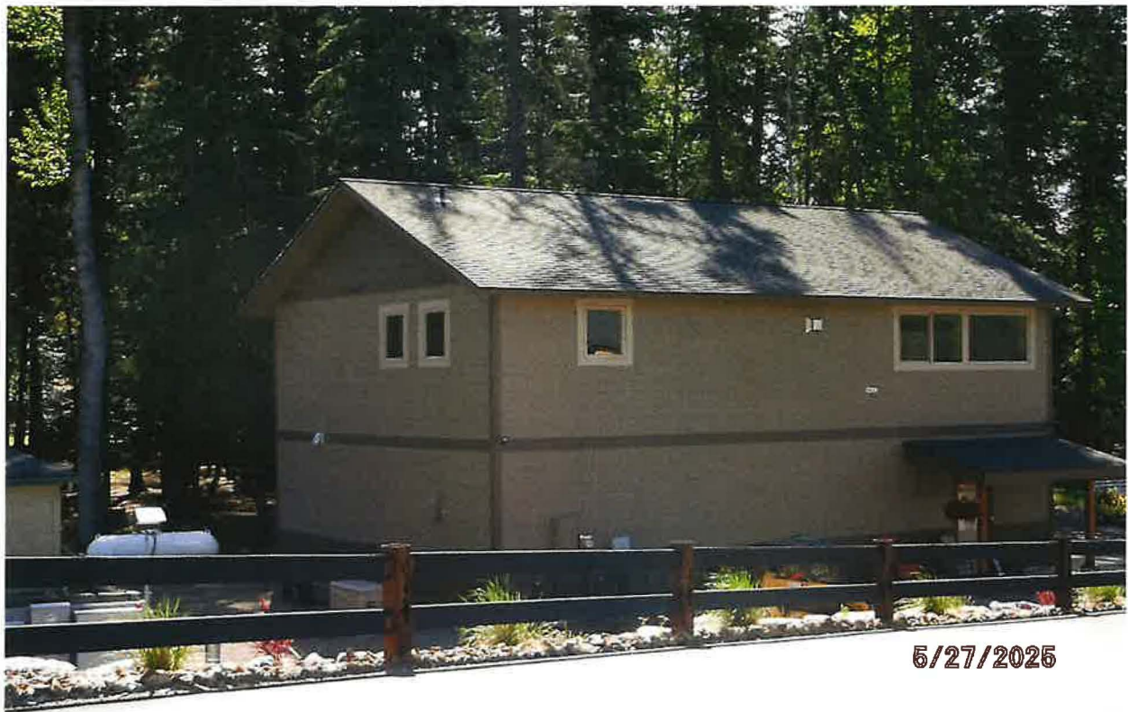
DOMESTIC POU – CARETAKER RESIDENCE (UPSTAIRS) / SHOP & PUMP STATION (DOWNSTAIRS)
