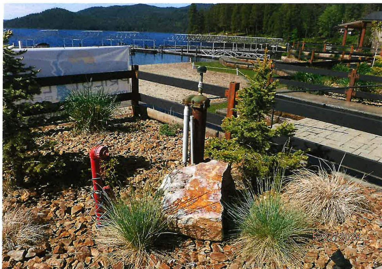
POD – 6-INCH CASED WELL 97-89-N-32-1
