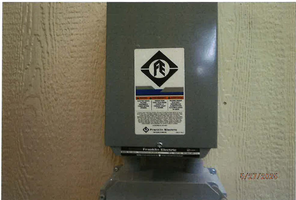
DIVERTING WORKS – 5 HP FRANKLINE ELECTRIC PUMP MOTOR
