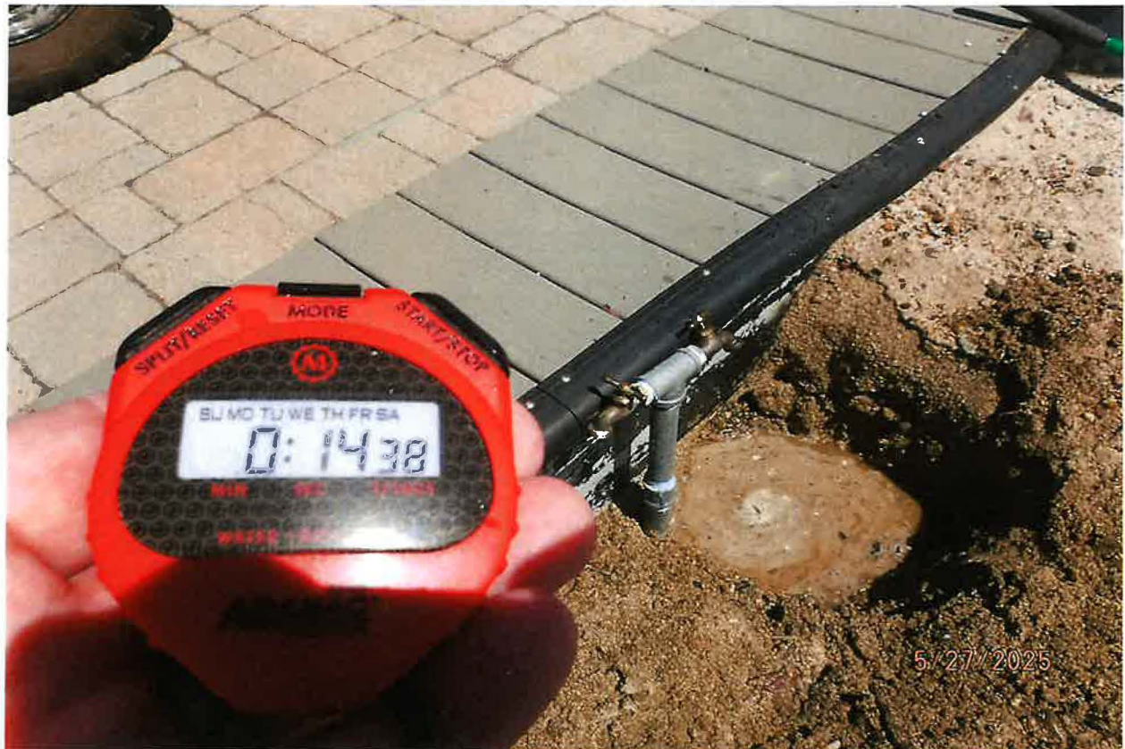
5 GAL BUCKET MEASUREMENTS TAKEN FROM HYDRANT LOCATED AT LAKE FRONTAGE
