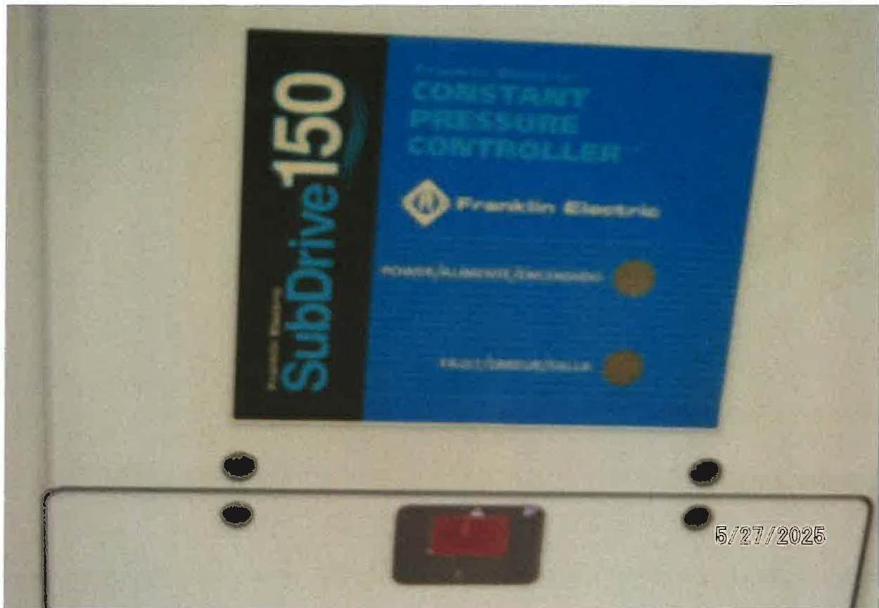
FRANKLIN ELECTRIC – SUBDRIVE 150 CONSTANT PRESSURE PUMP CONTROLLER
