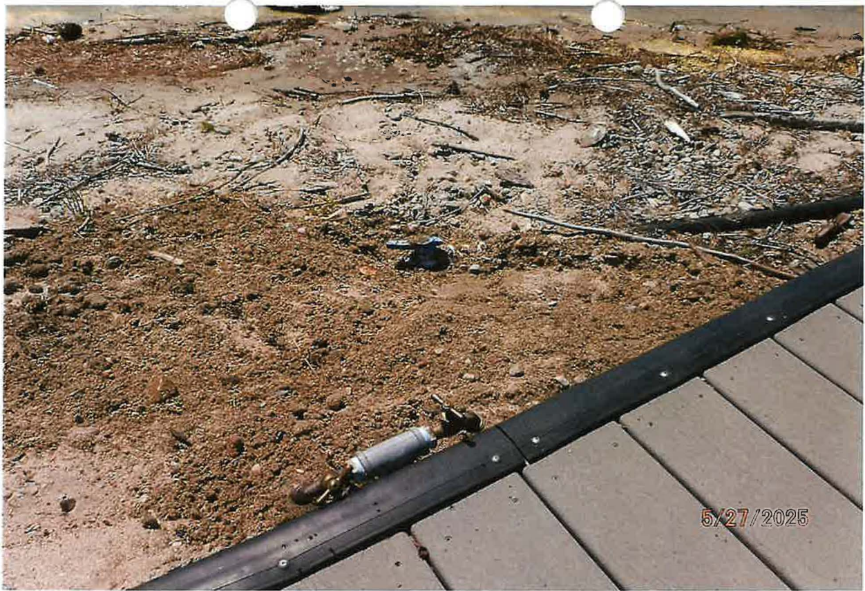
CONVEYANCE SYSTEM – 2-INCH MAIN LINE TO SHORE AND DISTRIBUTION TO 82 EA PRESSURIZED IRRIGATION SPRINKLER ZONES
