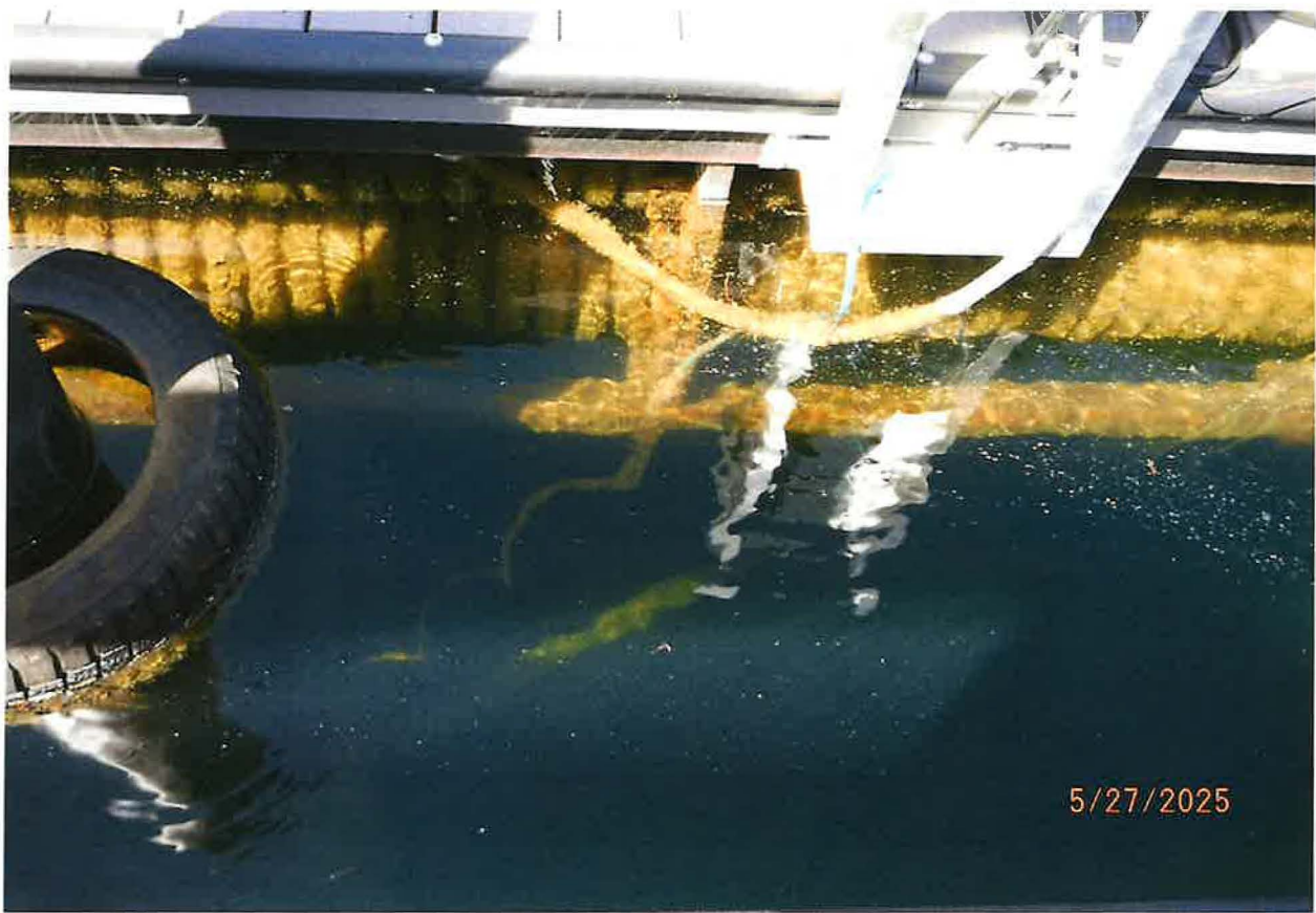
POD – DOCK MOUNTED INTAKE PIPE WITH SUBMERSIBLE 3 HP PUMP MOTOR
