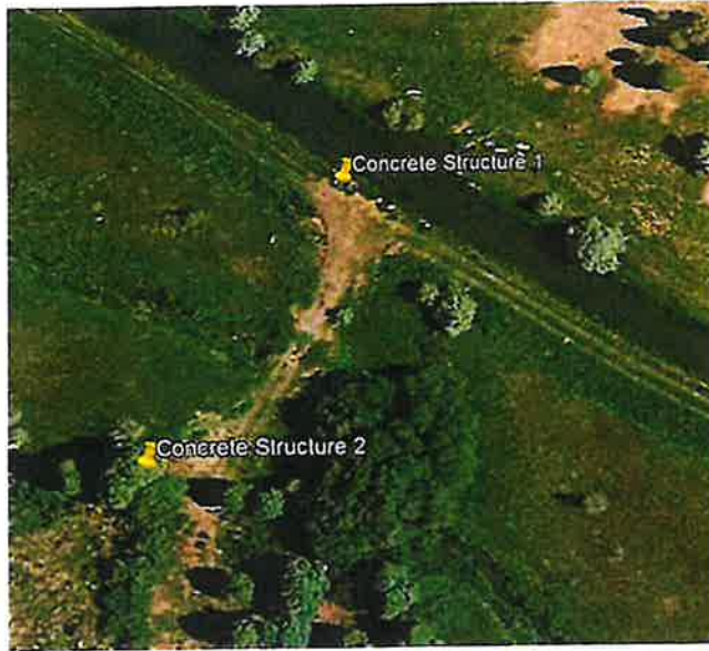
Concrete structures near the Soda Canal.
