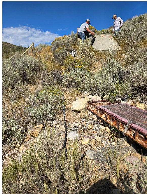
Figure 6: Black hose connected to the cistern and reaches stock troughs below the cistern.
