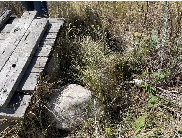
Figure 2: Cistern with wooden lid and inlet PVC pipe visibly protruding from the ground with a connecting hose into the cistern.
