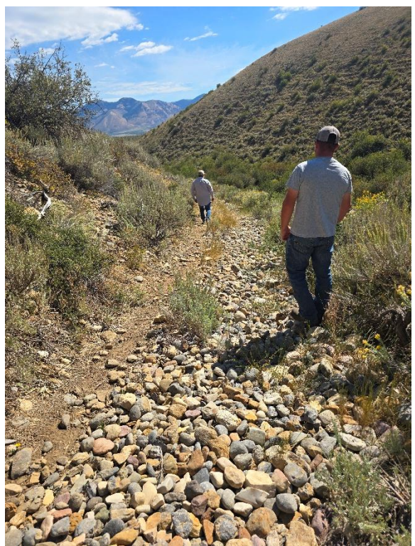
Figure 9 & 10: Roadway leading from the POD to the claimed POU shows a distinct depression on the right side that is filled with rocks. Possible runoff system. Under this area is where the diversion works is buried leading towards claimed POU.
