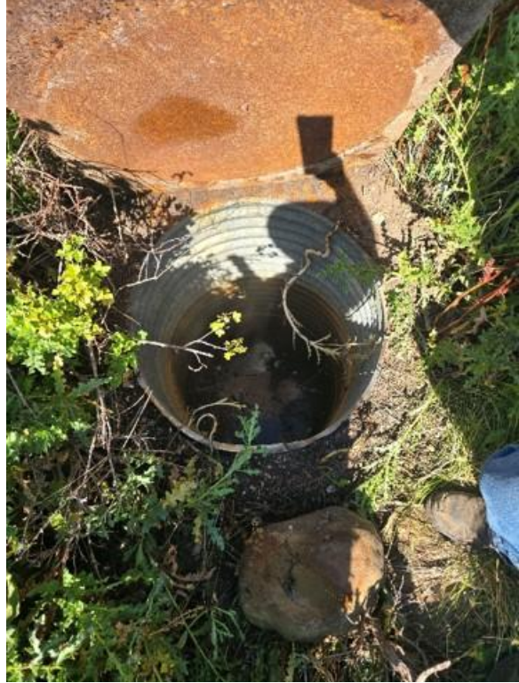
Figure 8: Actual POD used to collect water. Unable to see inlet and outlets due to current water inside collection container.
