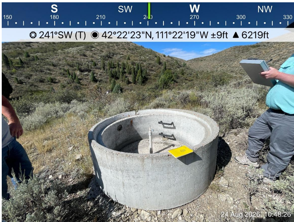
Figure 13: Cement stockwater trough.
