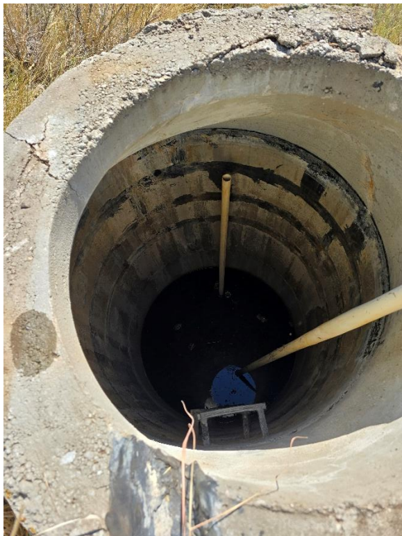
Figure 5: Interior of cistern.
