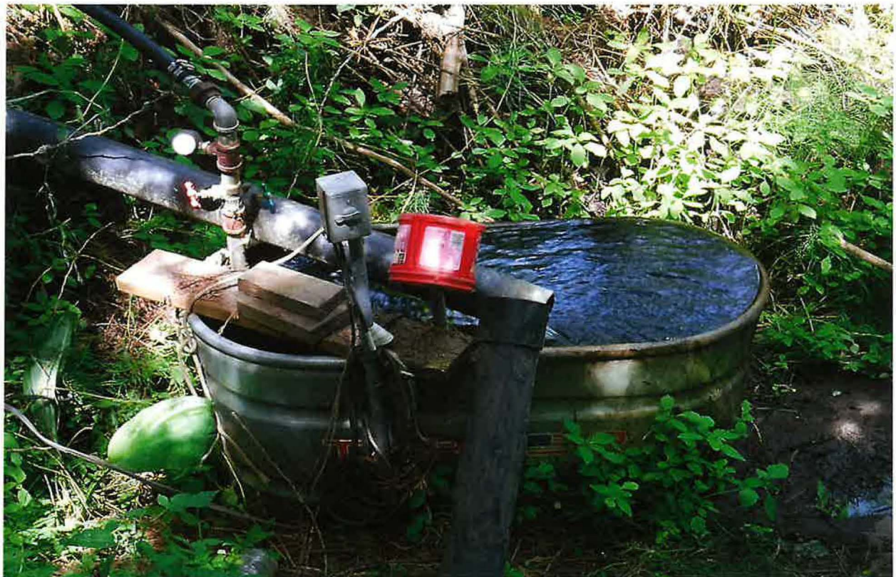
DIVERSION TO STORAGE – SPRING WATER FROM SPRING FIELD & OVERFLOW DISCHARGE FROM STORAGE POND CAPTURED AND PUMPED BACK TO POND
