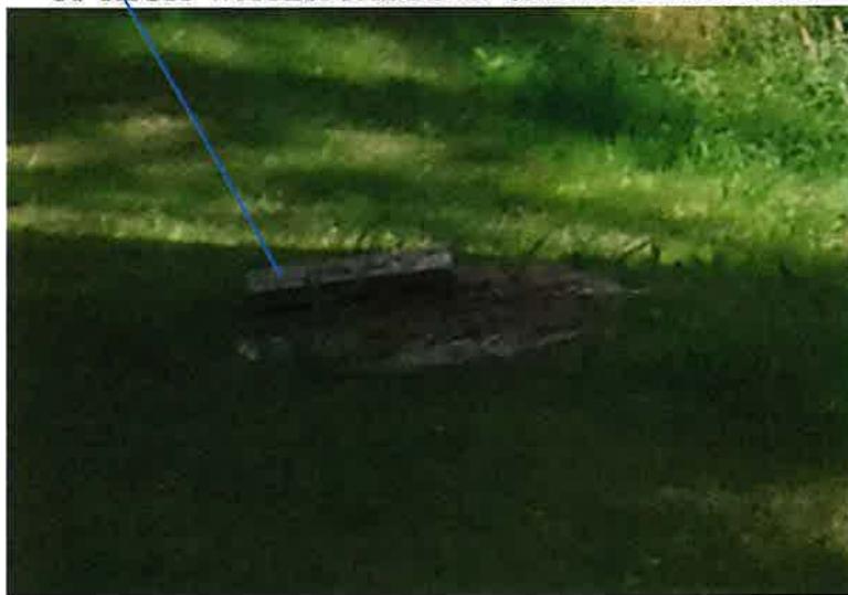
SHALLOW HAND DUG WELL USED FOR DEFERABLE DOMESTIC USE – INDICATIVE OF HIGH-WATER TABLE IN SMALL DRAINAGE
