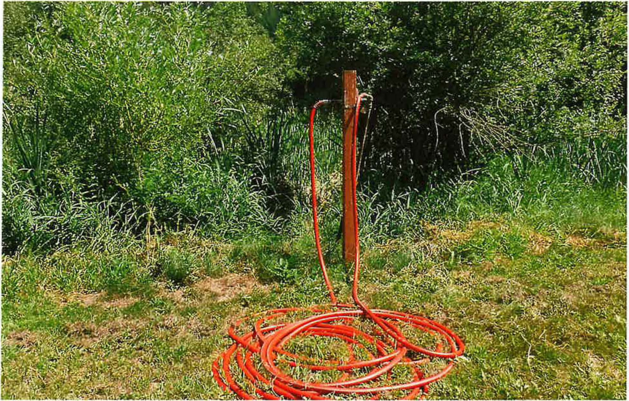
IRRIGATION FROM STORAGE – STORAGE POND WATER PUMPED VIA POLY PIPE TO IRRIGATION RISER PIPE CONNECTING HOSE AND SPRINKER FOR ROTATIONAL IRRIGATION WATERING
