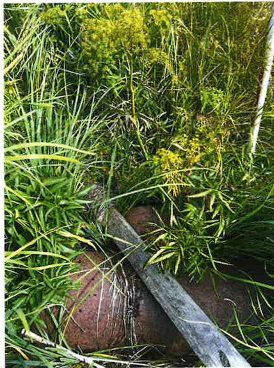
Figure D: Example of tee pipe that lets water out of the ditch onto the field.
