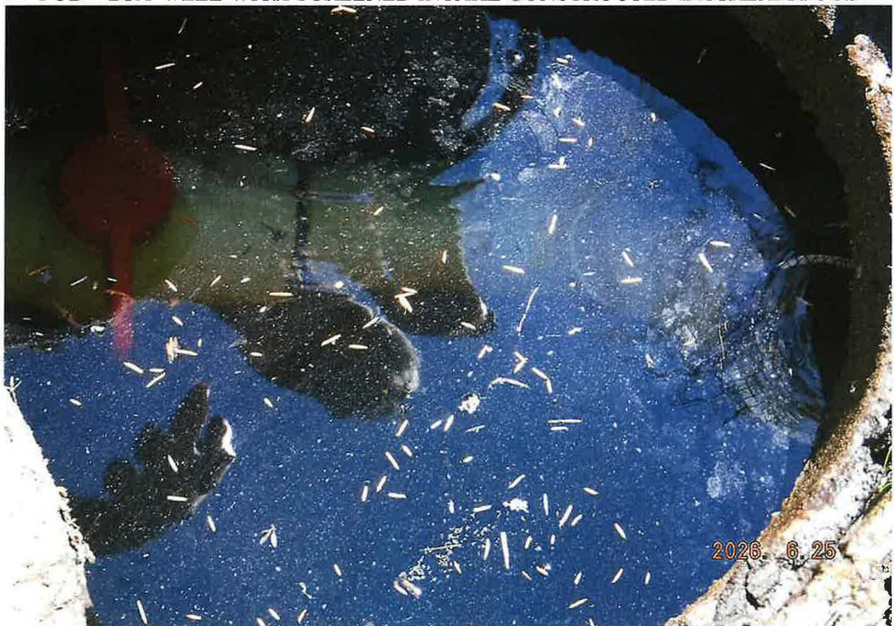
INTERIOR DRY WELL – MESH SCREEN ON 4-INCH PVC PENSTOCK PIPELINE TO POU
