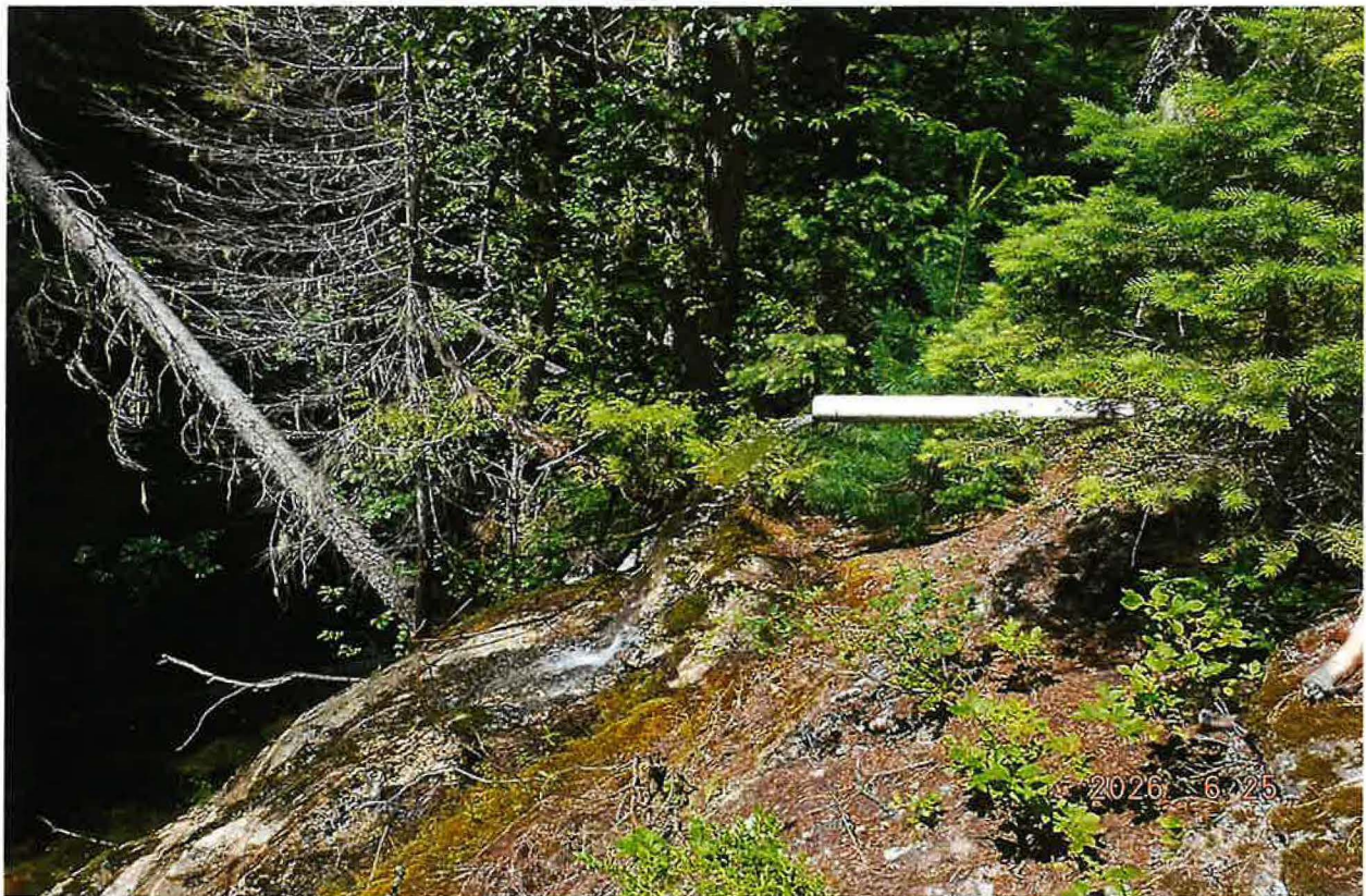
6-INCH DISCHARGE FROM MICRO-HYDRO RETURNS FLOW TO FALL CREEK SPLASHING DOWN ROCK CREEK FRONT
