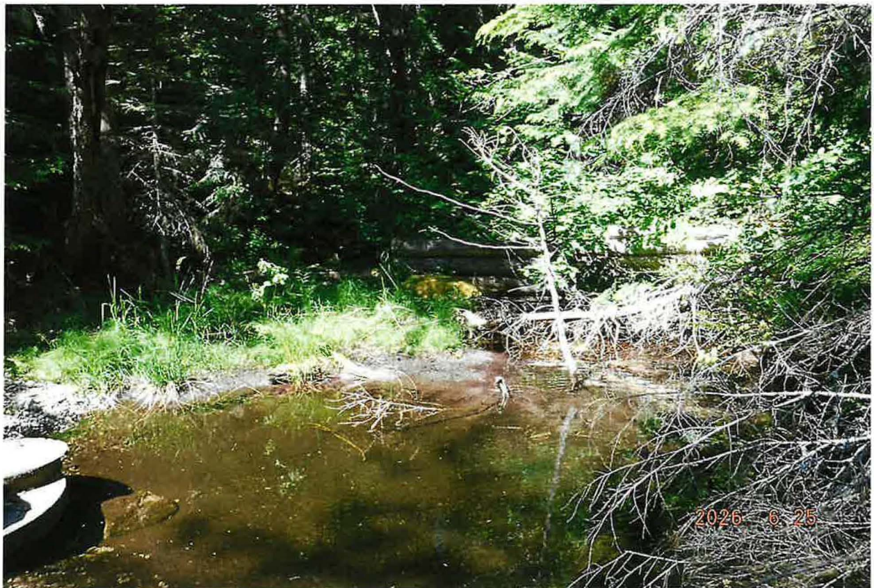
POD – UNNAMED STREAM DIVERSION USING DRY WELL CONSTRUCTED IN SMALL POOL AREA OF STREAM
