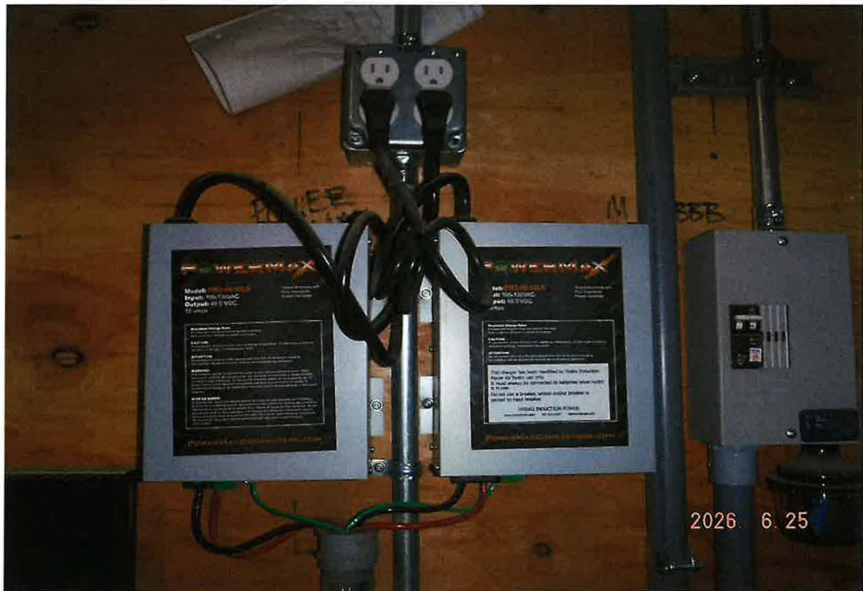
2EA POWERMAX CONVERTERS MODEL PM3-48-18LK
