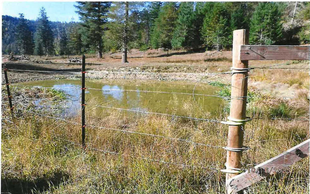
POD AND POU – LOWER SOUTHWESTERN STORAGE POND AND EARTHEN BANK POD WHICH IMPOUNDS UNNAMED STREAM FLOW FROM UPPER POND
