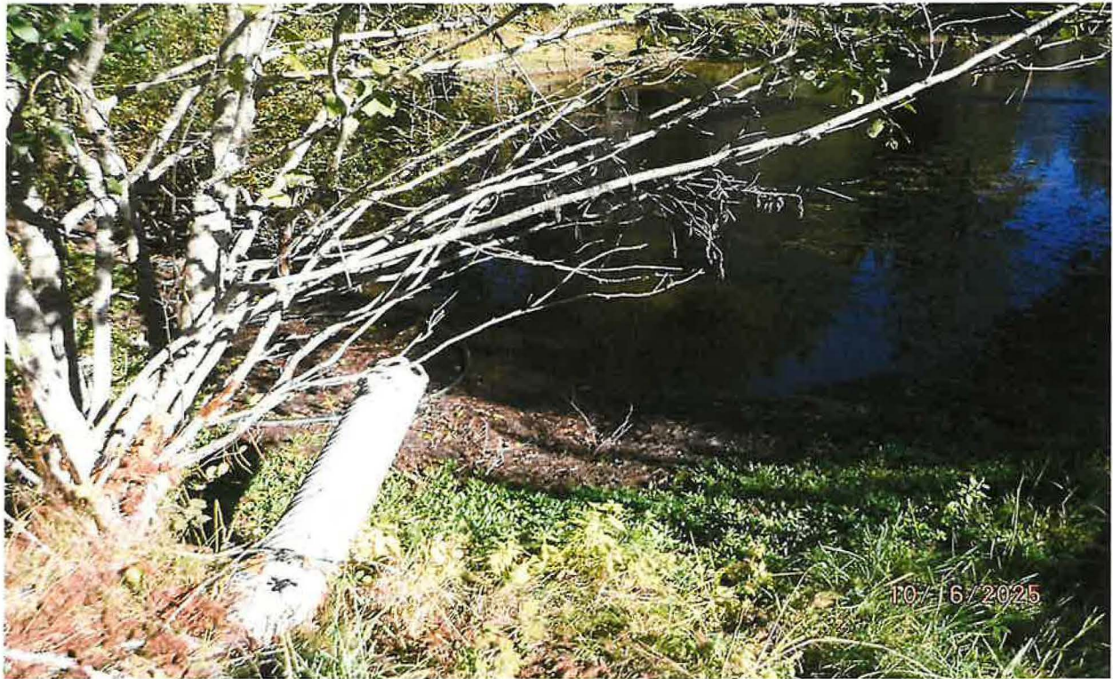
8 INCH STEEL OVERFLOW DISCHARGE PIPE FROM NORTHEASTERN POND BECOMES START OF UNNAMED STREAM SOURCE WHICH FEEDS LOWER SOUTHWESTERN POND – LATE FALL LOW WATER LEVELS RESULT IN DRY STREAM BED
