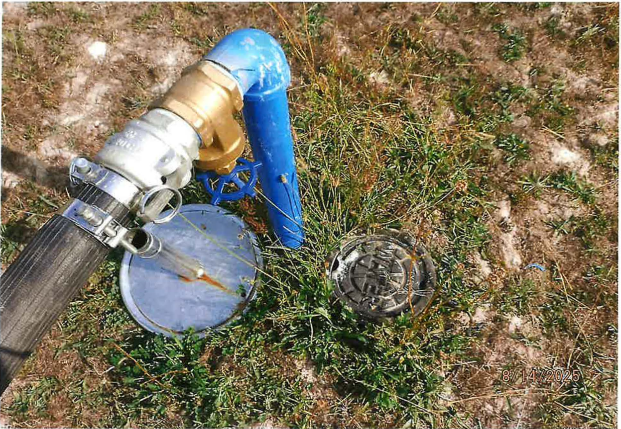
IRRIGATION POU – LAST IRRIGATION RISER PIPE CONNECTED TO BIG WHEEL SPRINKLER
