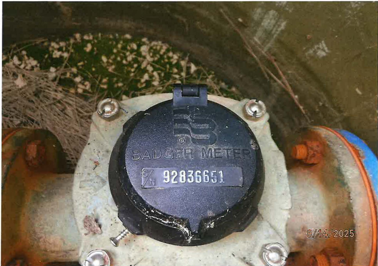
BADGER METER – RECORDALL FLANGED VELOCITY STYLE FLOW METER S/N 92836651 INSTALLED PRIOR TO FIRST IRRIGATION RISER
