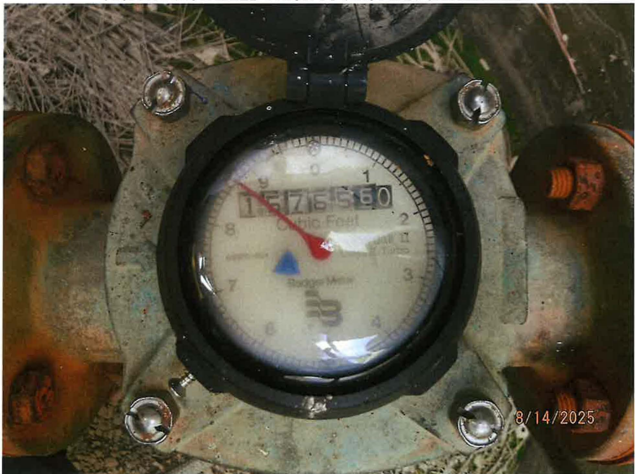
BADGER METER – RECORDALL FLANGED VELOCITY STYLE FLOW METER S/N 92836651 INSTALLED PRIOR TO FIRST IRRIGATION RISER
