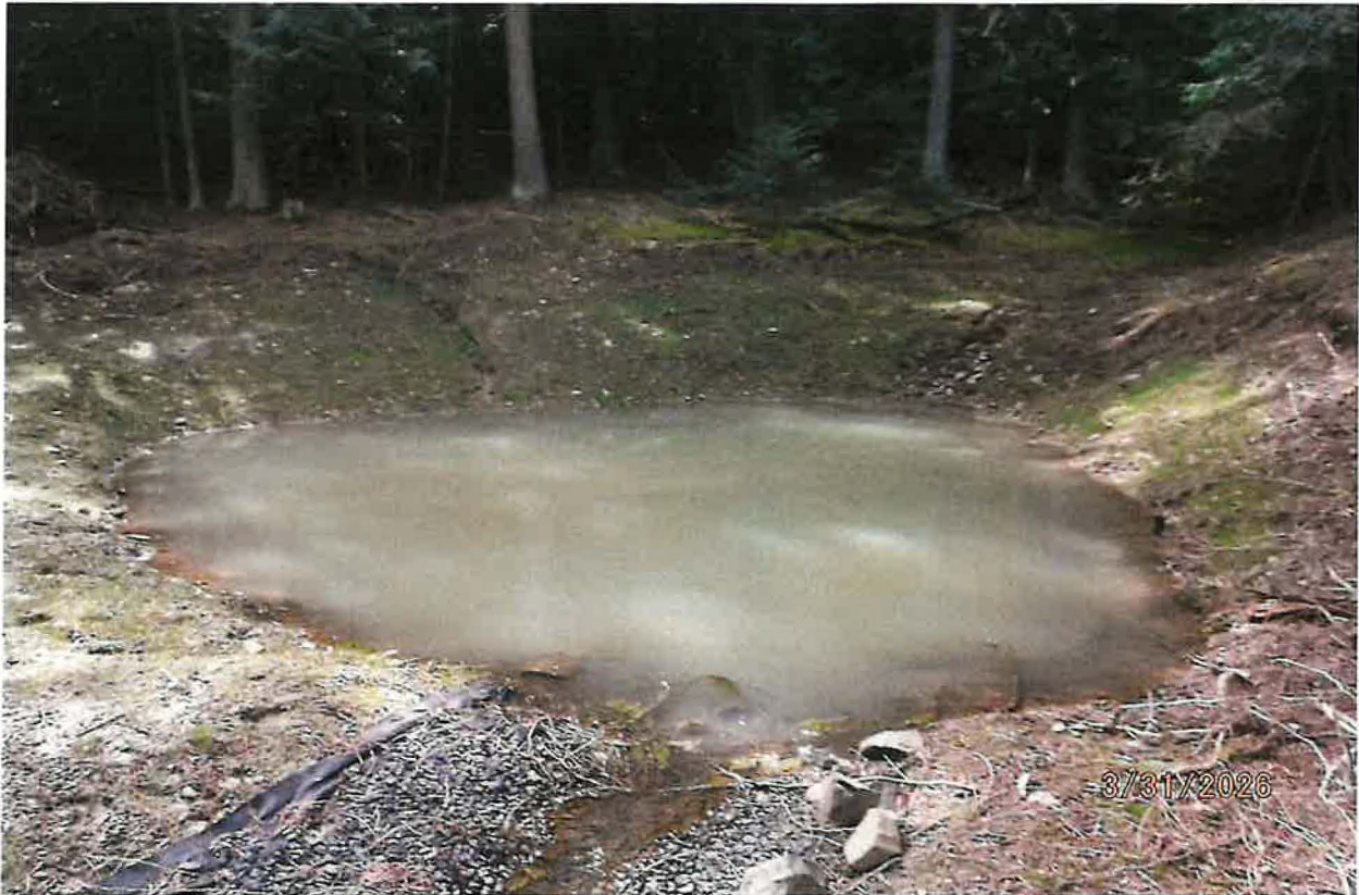
STORAGE POND SYSTEM IS 6-8 FT MAX DEPTH; NO IRRIGATION FROM STORAGE BENEFICIAL USE DEVELOPED FROM SMALL POND
