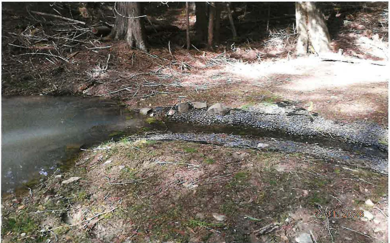
POD – SKID TRAIL EMBANKMENT WITH GRAVEL OVERFLOW CHANNEL
