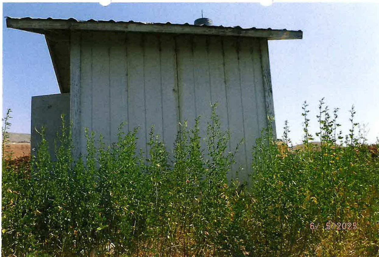
POD – PUMP STATION
