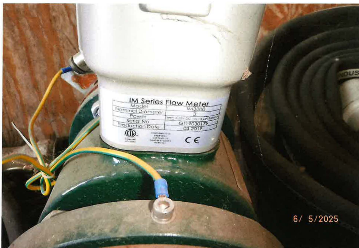
IM SERES FLOWMETER – MODEL IM3000, S/N GT19030179 WITH MFD 3/2019
