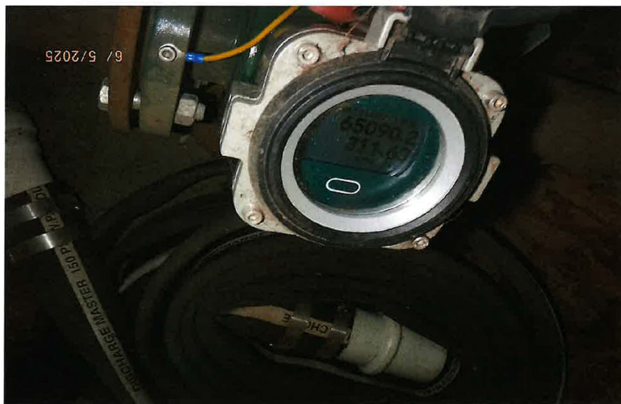
FLOW METER DIGITAL READOUT – 311 GPM ILLUSTRATED AS SYSTEM WAS STILL STABILIZING
