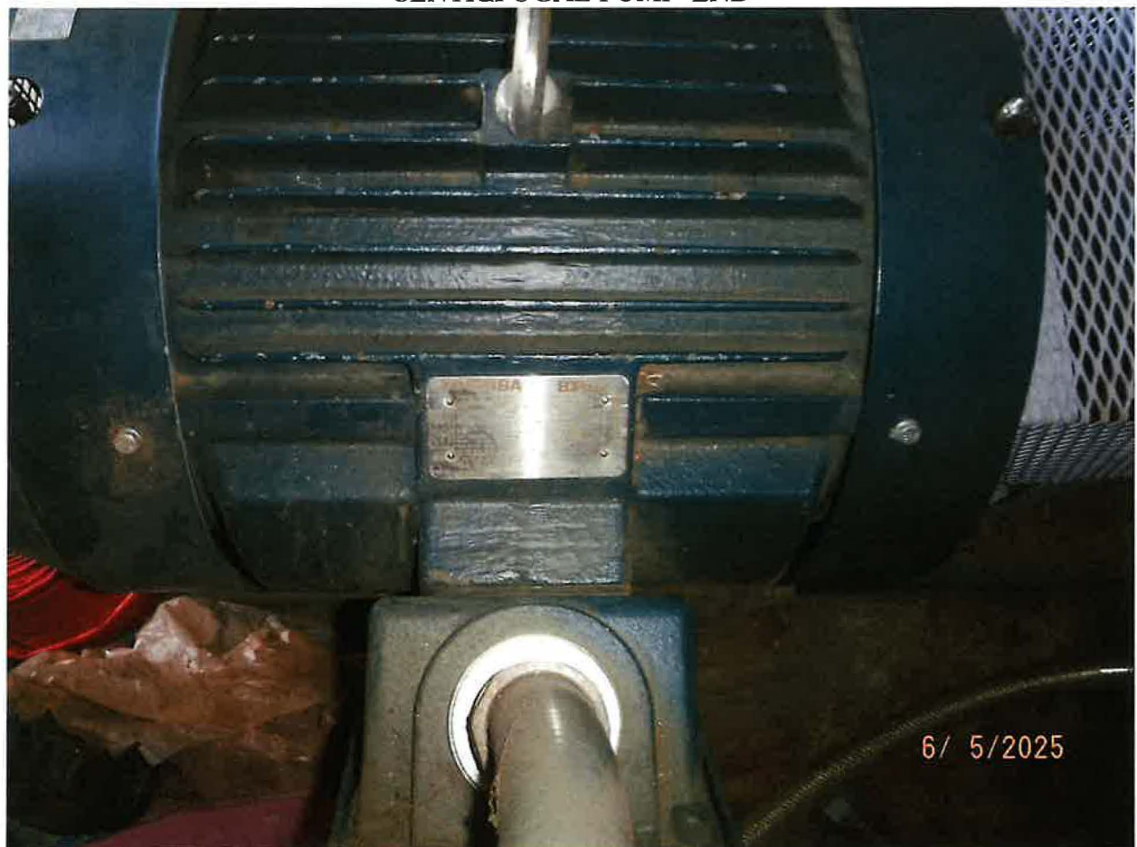
DIVERTING WORKS – 75 HP TOSHIBA MOTOR SD-75H-36-TEFC WITH 36TS FRAME & CENTRIFUGAL PUMP END
