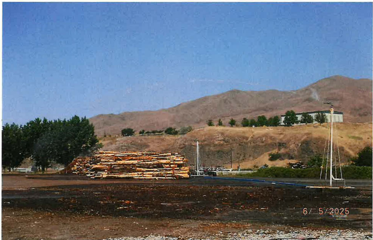
INDUSTRIAL POU – LOG DECK WATERING EXCESS WATER SHEET RUNS NORTH ACROSS YARD ENTERING A DRAIN DITCH WHICH ROUTES TO AN ARMY CORP SETTLING LAGOON ON WESTERN SIDE OF POU
