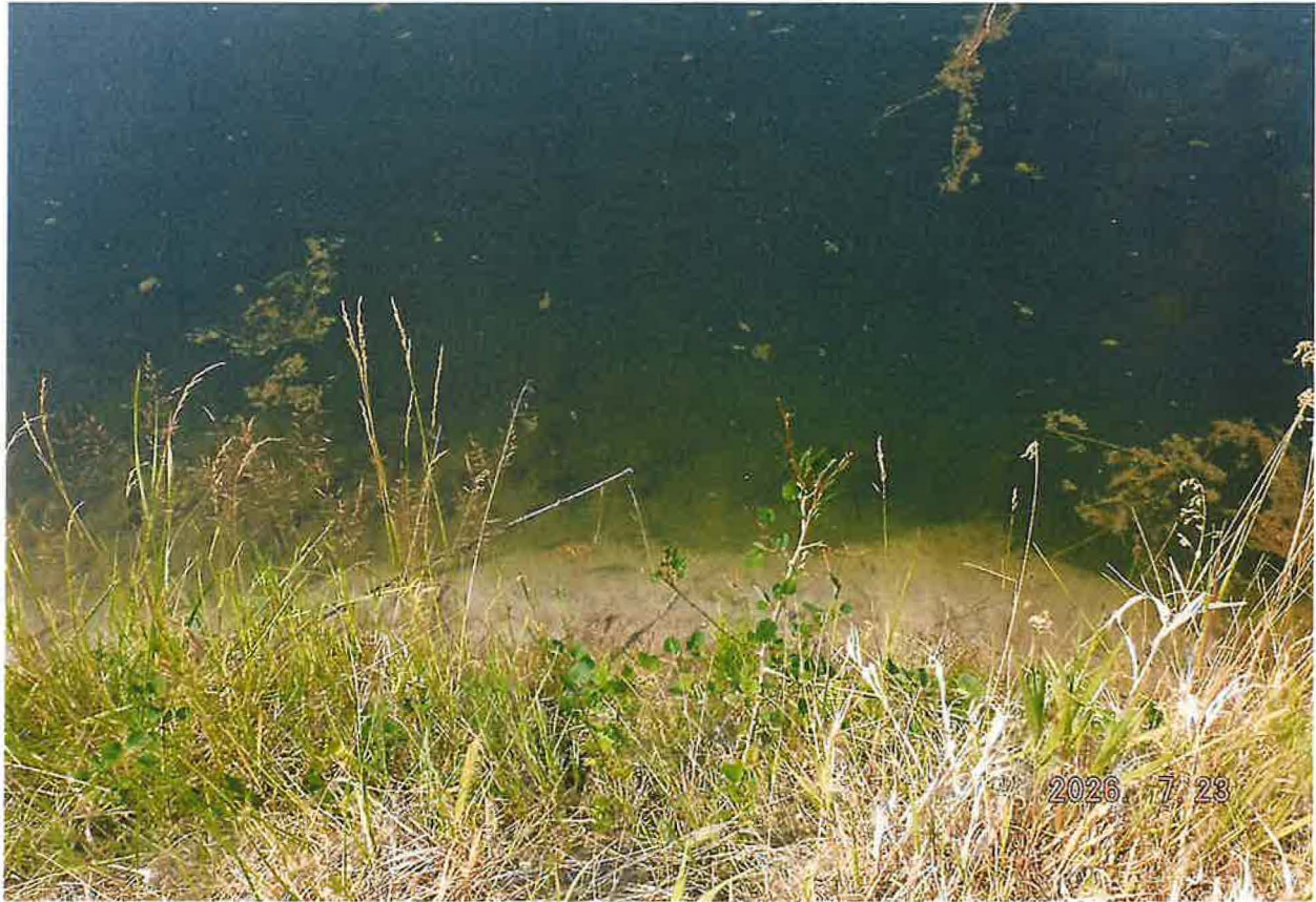
STEEP EMBANKMENT SLOPE
