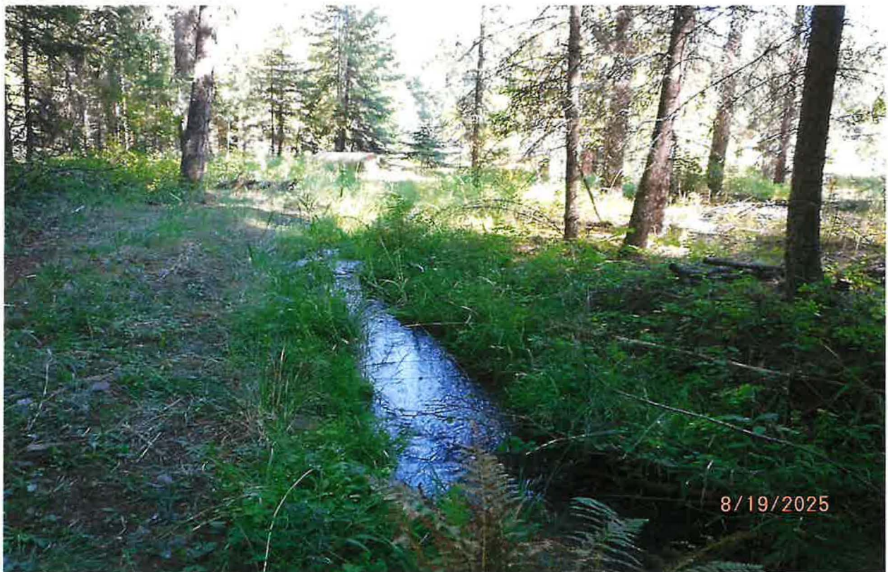
CONVEYANCE DITCH DOWN REACH OF CONFLUENCE WITH UNNAMED STREAM
