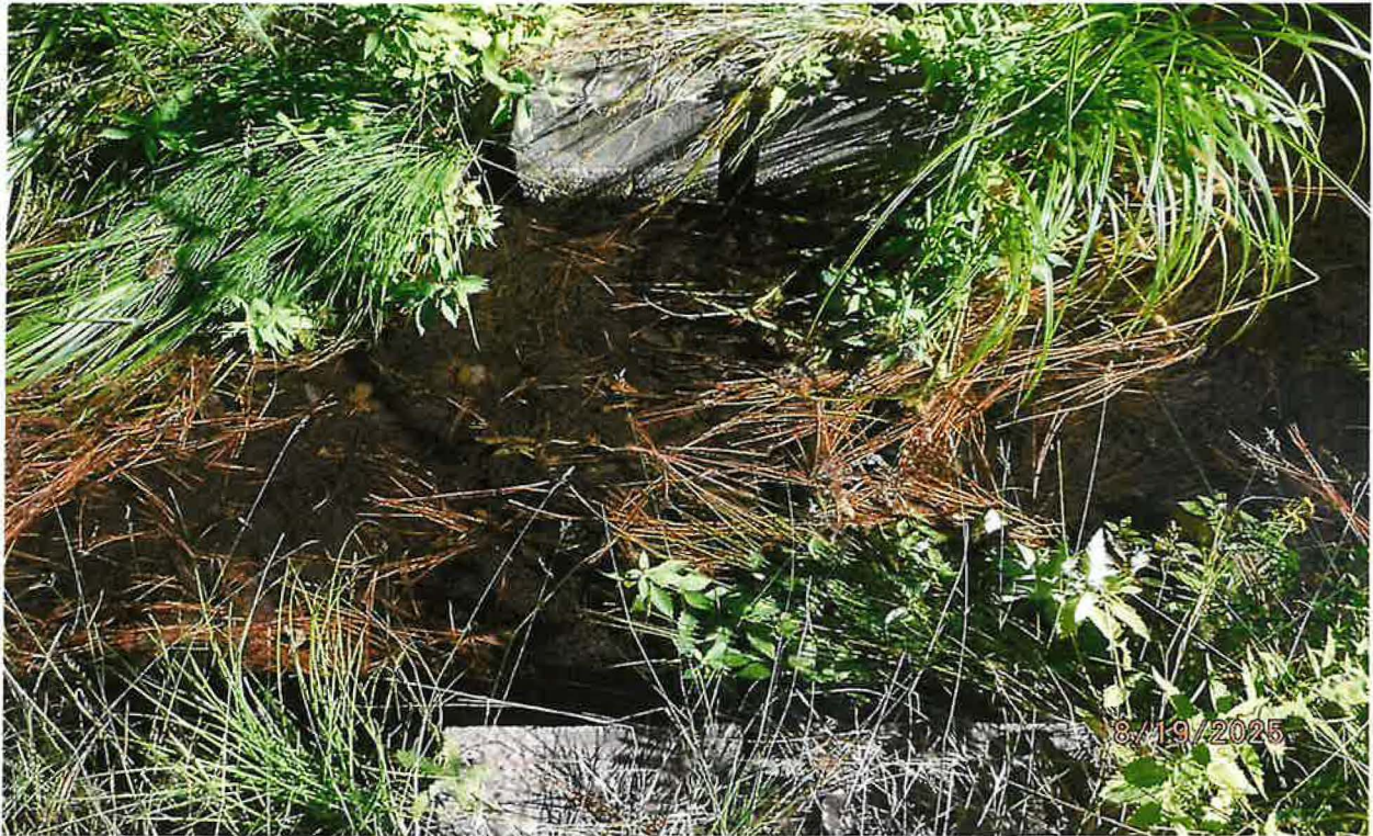
RECREATION POU – PRIMARY OVERFLOW DEVICE POND #5 – 2-FT WIDE CHANNEL BANDED WITH CONCRETE ALLOWS OVERFLOW DISCHARGE TO FLOW IN EARTHEN CHANNEL A SHORT DISTANCE INTO A FIELD WHERE IT SINKS (NORTHWEST BANK OF POND)
