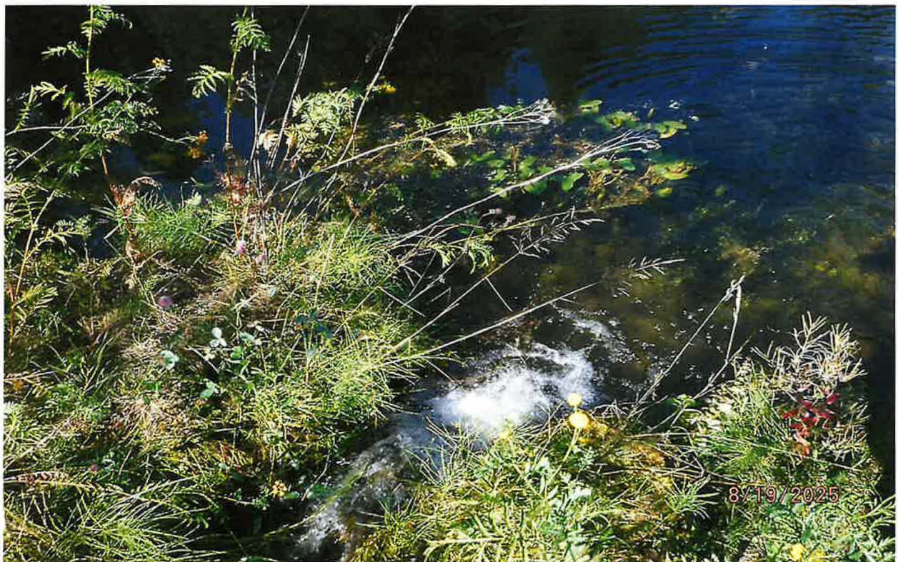
RECREATION POU – OVERFLOW NATURAL CHANNEL DISCHARGES FROM POND #2 TO POND #3 IN SERIES
