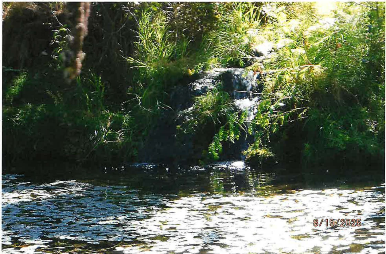
RECREATION POU – OVERFLOW NATURAL CHANNEL DISCHARGES FROM POND #4 TO POND #5 IN SERIES
