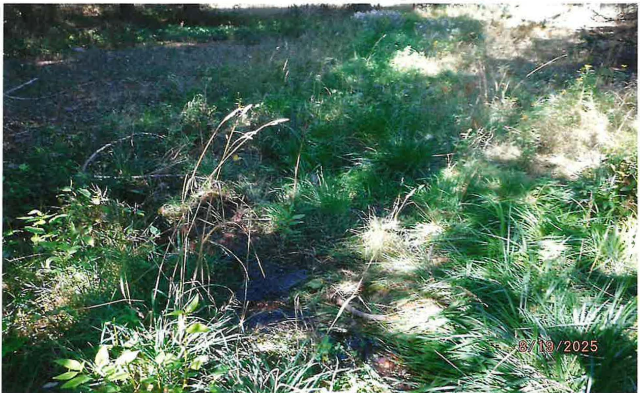
END OF OVERFLOW WATER FROM POND #5 SINKING TO GROUND PRIOR TO REACHING TWENTY MILE CREEK
