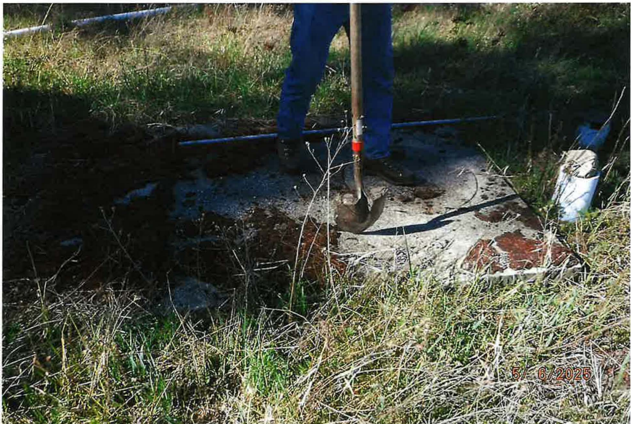
POD – SPRING WITH DRAIN TILES FILLING CONCRETE CISTERN
