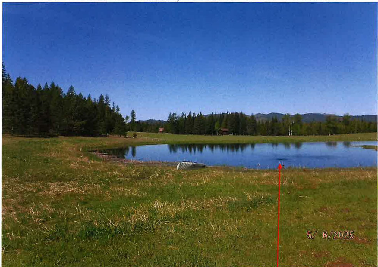
STORAGE POU – RIFFLE IN POND IS THE LOCATION OVERFLOW DIVERSION TO STORAGE PIPELINE INFILLS TO POND
