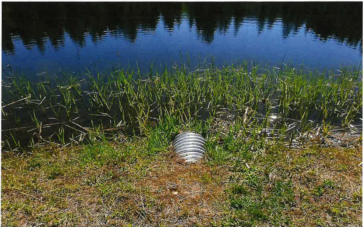
8-INCH OVERFLOW DISCHAGE CULVERT ALONG WESTERN EARTHEN DAM/DIKE FOR POND
