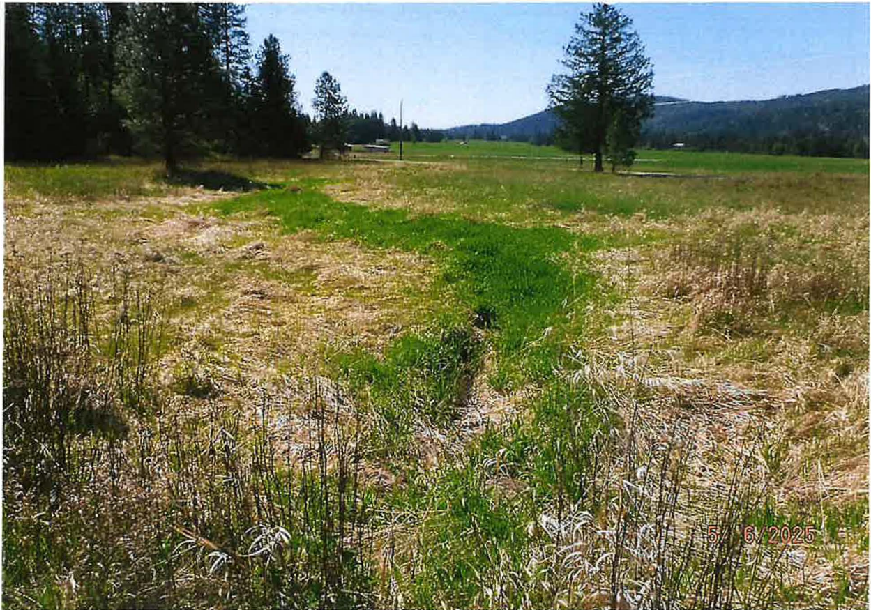
UNNAMED STREAM FLOWS IN CHANNEL WITH OVERFLOW DISCHARGING THROUGH METAL CULVERT ON SOUTHERN PART OF STORAGE POND
