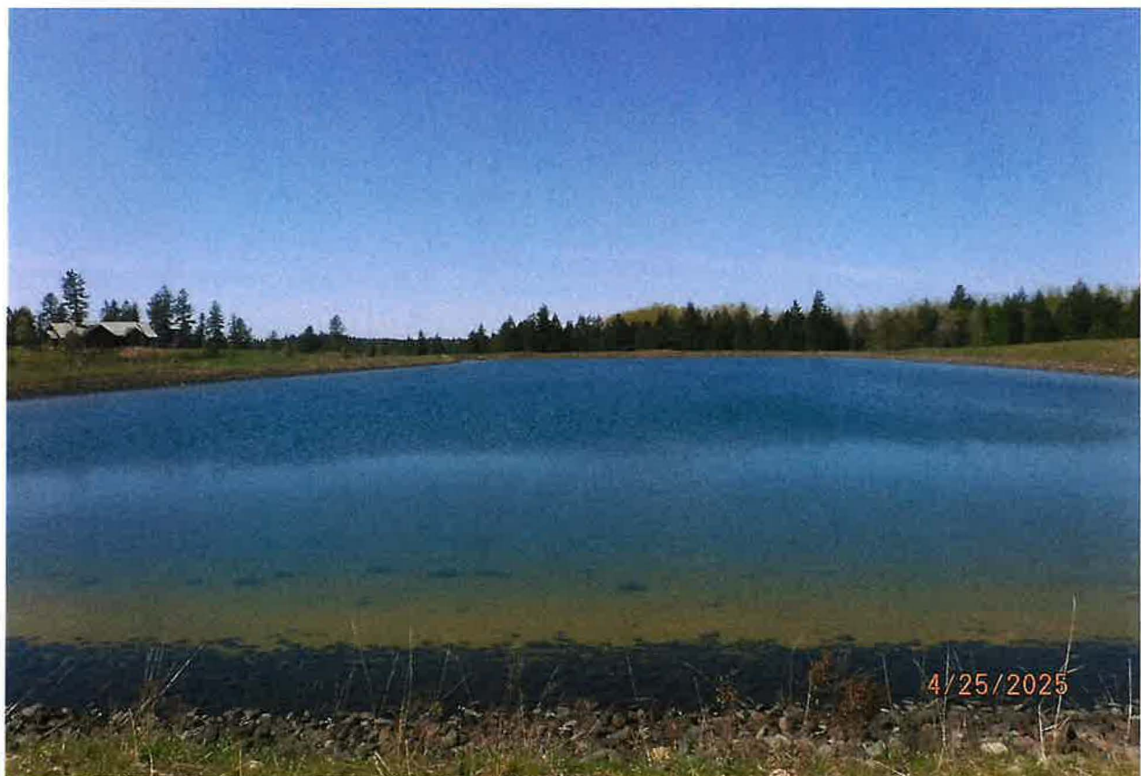
POU – 3.02 ACRE MUNICIPAL STORAGE POND
