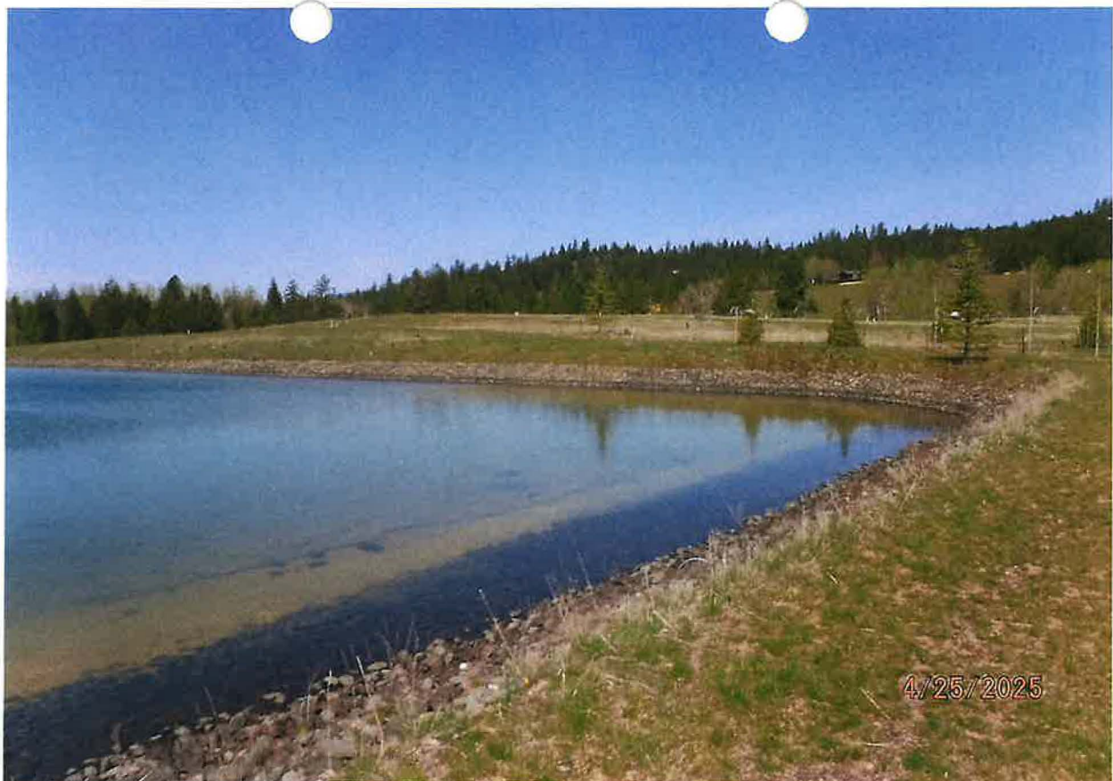
STORAGE RESERVOIR (POND) IS LINED TO MITIGATE SEEPAGE LOSS OF IMPOUNDED LAKE WATER
