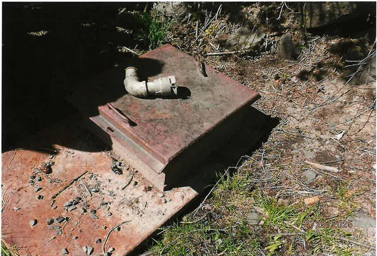
POD – VAULTED ACCESS TO MAIN PIPELINE WHICH HOUSES 2EA 4" PVC PIPELINES, ONE PER PUMP – ACCESS TO REPLACE/WORK ON PUMPS
