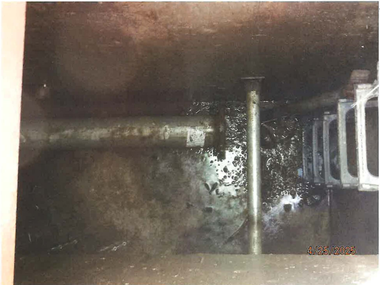
POD – VAULTED ACCESS TO MAIN PIPELINE WHICH HOUSES 2EA 4" PVC PIPELINES, ONE PER PUMP – ACCESS TO REPLACE/WORK ON PUMPS
