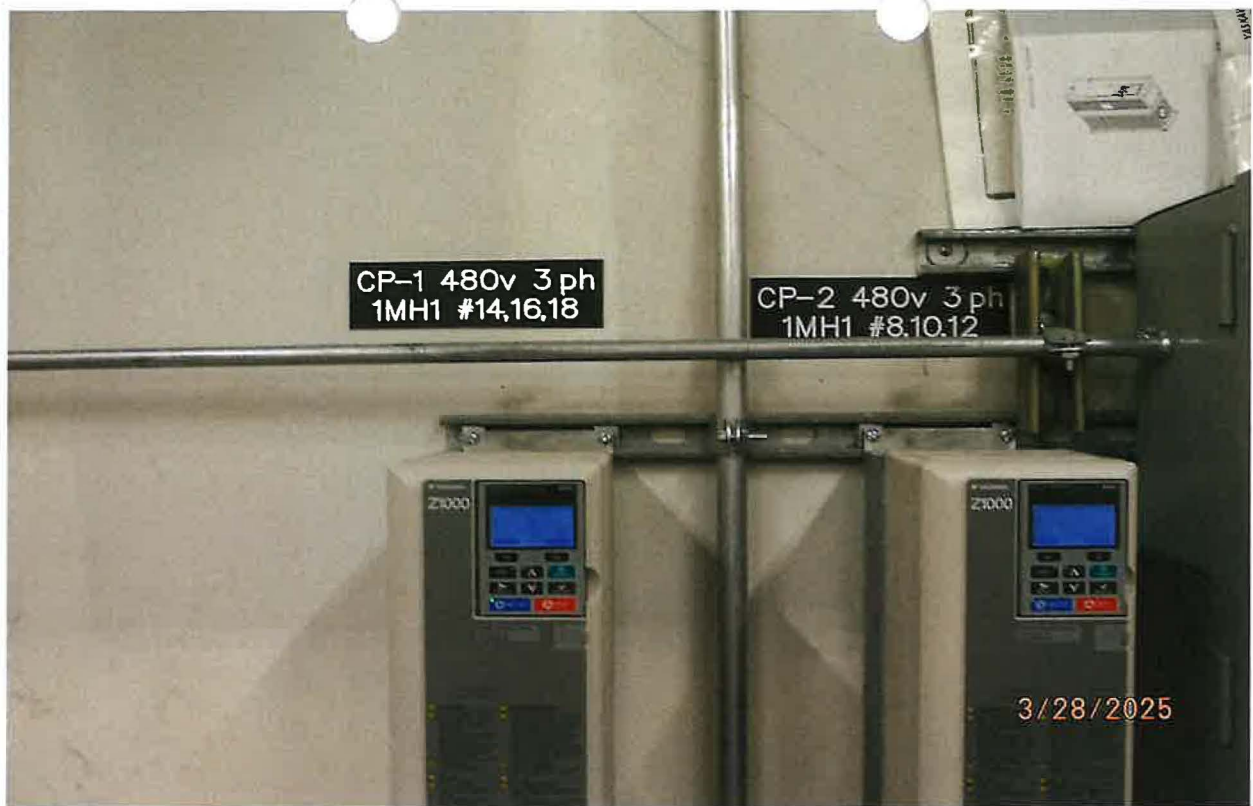
2EA 10 HP LOOP PUMP (CP-1 & CP-2) CONTROL PANELS
