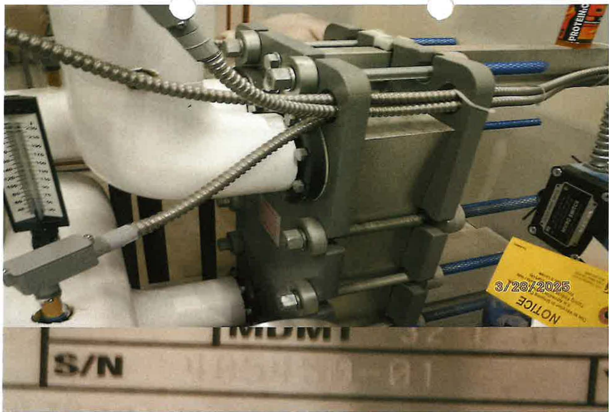
HEAT EXCHANGER – ARMSTRONG BRAND, MODEL NO. A22H-150-70-1000, S/N 405450-01
