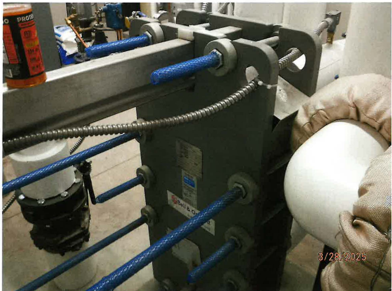
HEAT EXCHANGER – ARMSTRONG BRAND, MODEL NO. A22H-150-70-1000, S/N 405450-01
