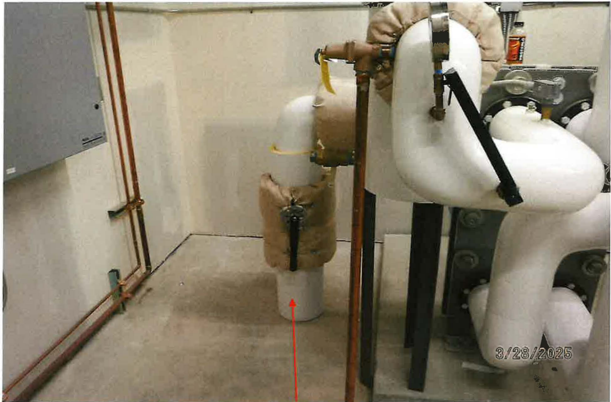
WATER CONVEYANCE SYSTEM – INFLOW FROM DIVERTING WELL TO HEAT EXCHANGER
