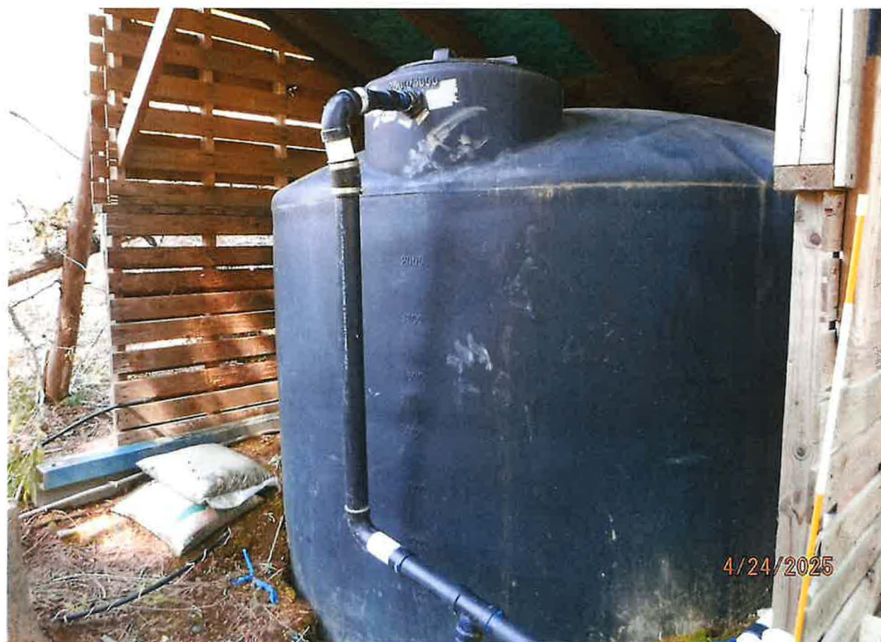
2,500-GAL STORAGE RESERVOIR SERVES WATER USE FOR WATER RIGHTS 92-11089AND 92-11097
