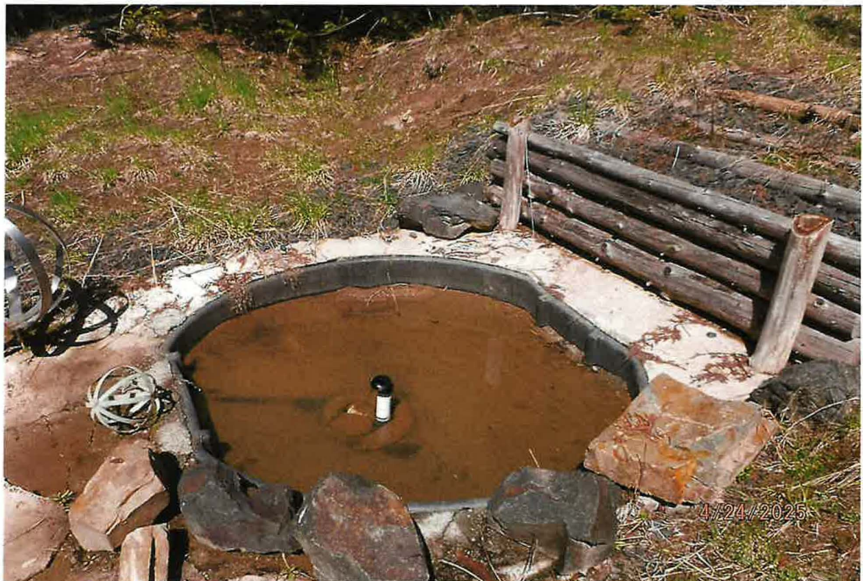
POD – EASTERN MOST POD, RUBBER MADE TUB INSTALLED IN SWALE TO COLLECT UNNAMED STREAM WATER; PUMPED TO STORAGE TANKS
