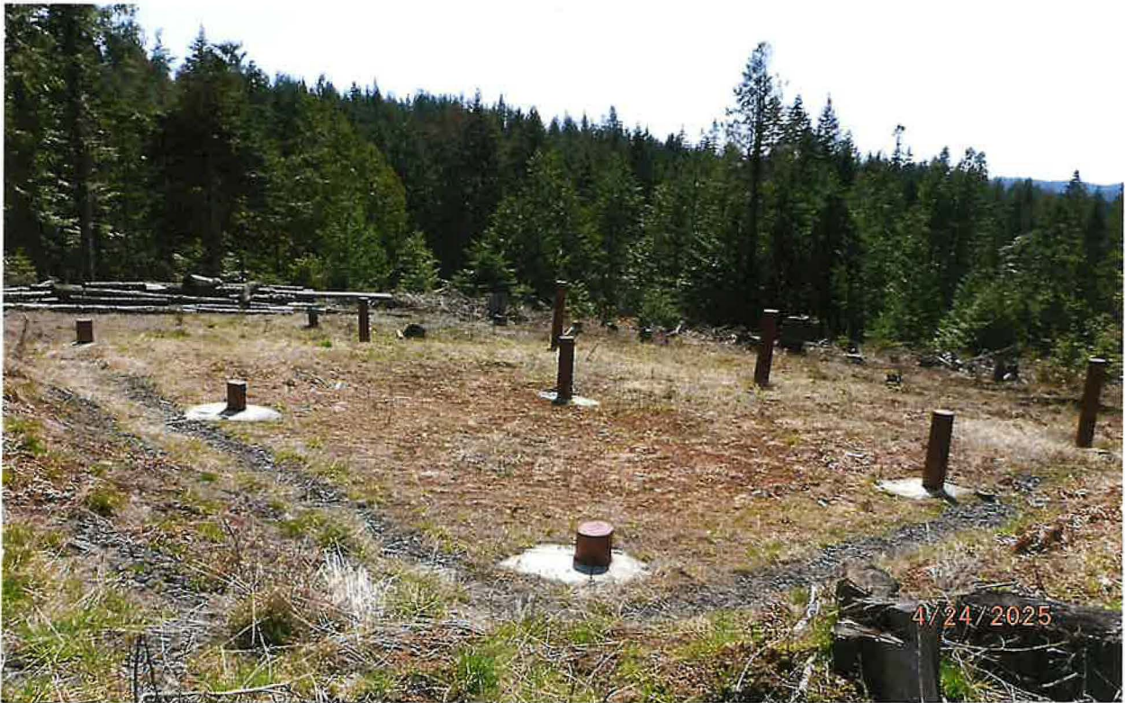
DOMESTIC POU – HOME SITE PREPARED FOR DEVELOPMENT WITH SERVICE LINE ROUTED TO CENTER OF PAD. DOMESTIC USE IS FOR A LIVE-IN RV ON-SITE WHILE CONSTRUCTING THE PRIMARY RESIDENCE
