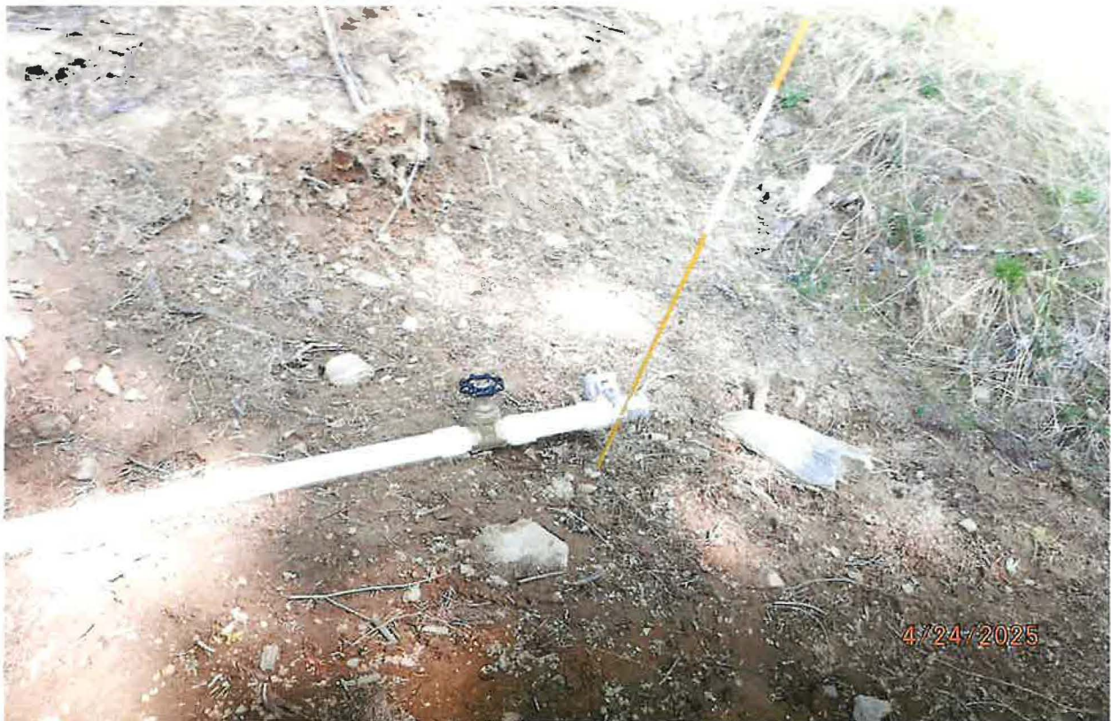
WATER FILL STATION FROM 2,500-GAL STORAGE TANK – PORTABLE TANKS FILLED FOR USE AT OFF-GRID RESIDENCES
