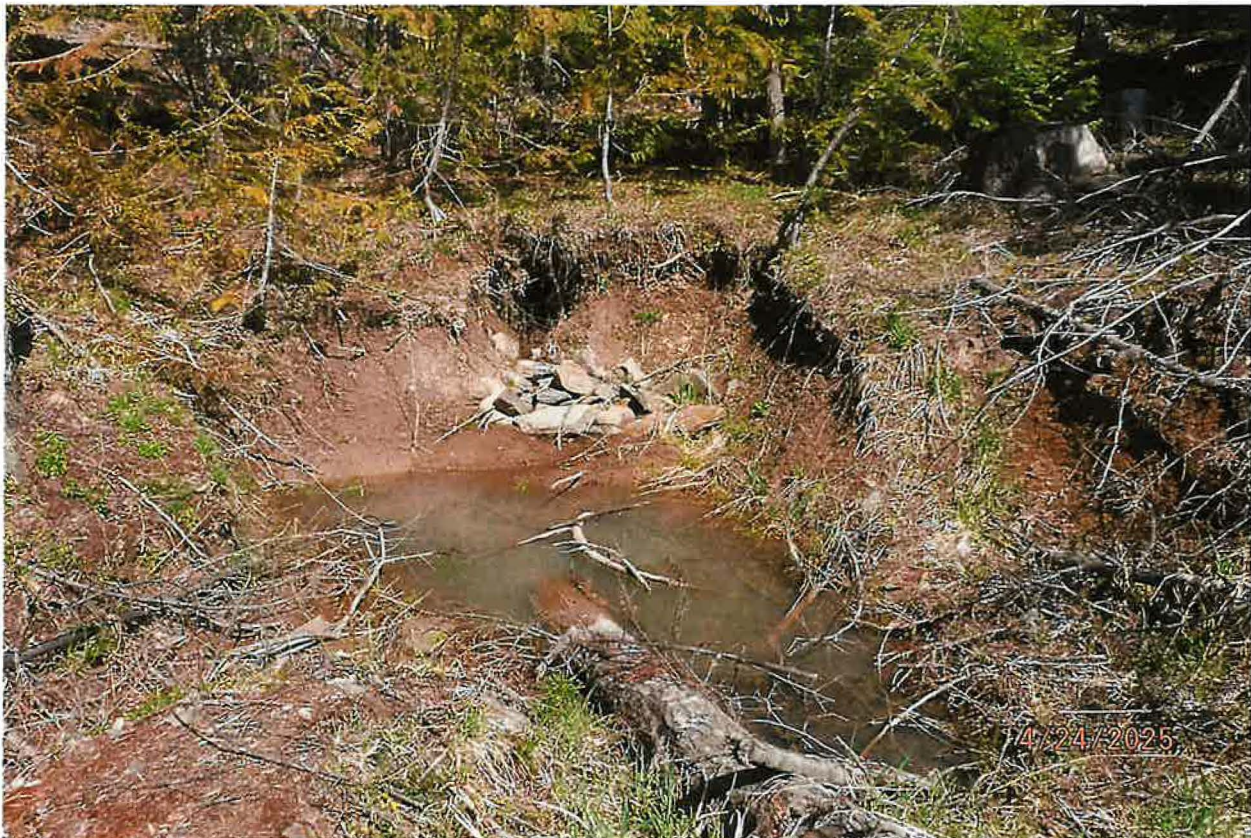
POD – WESTERN MOST POD, SMALL COLLECTION POOL DUG OUT TEMPORARILY CAPTURING STREAM WATER WHICH IS PUMPED TO STORAGE TANKS
