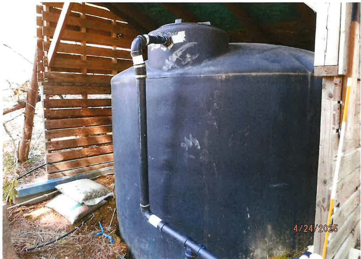
2,500-GAL STORAGE RESERVOIR SERVES WATER USE FOR WATER RIGHTS 92-11089AND 92-11097
