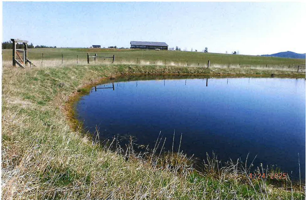
POD/POU – SPRING EXCAVATED POND WITH EARTHEN BERM DAM USED FOR RECREATION STORAGE & STOCKWATER STORAGE; NO INFLOW OR OUTFLOW FROM STORAGE POND
