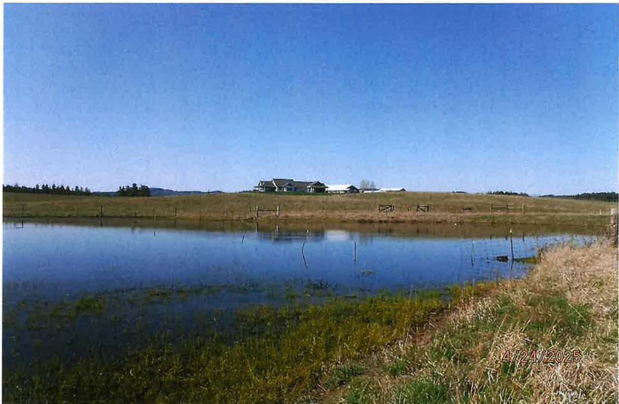
POU – STORAGE POND EARTHEN BERM DAM CONSTRUCTED ALONG WESTERN/NORHTERN/EASTERN RADIUS OF POND
