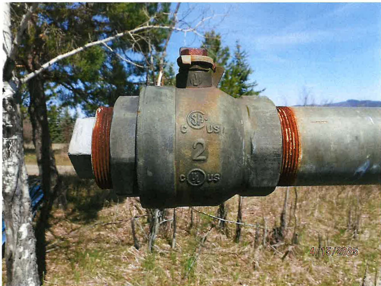
FIRE PROTECTION POU – 2-INCH FIRE TENDER FILL POINT
