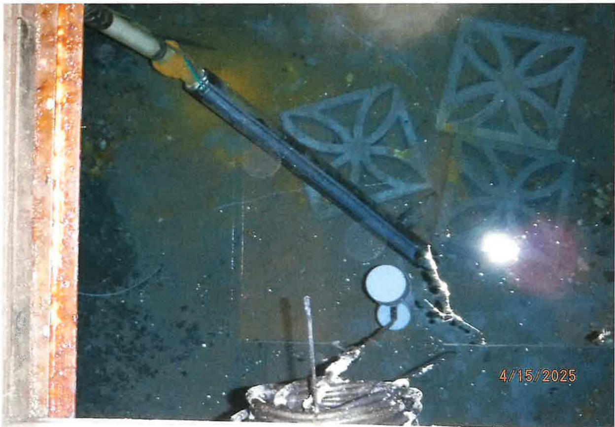
POD – VAULTED SPRING CISTERN – VIEW LOOKING IDOWN FROM ACCESS DOOR AT WATER & PUMP DIVERTING WORKS
