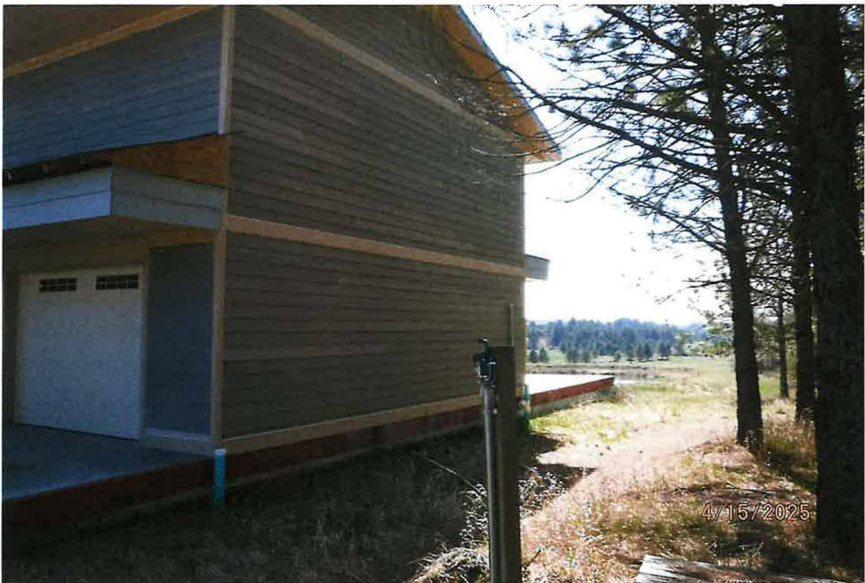
HYDRANT LOCATED AT MAIN RESIDENCE FOR DOMESTIC USE
