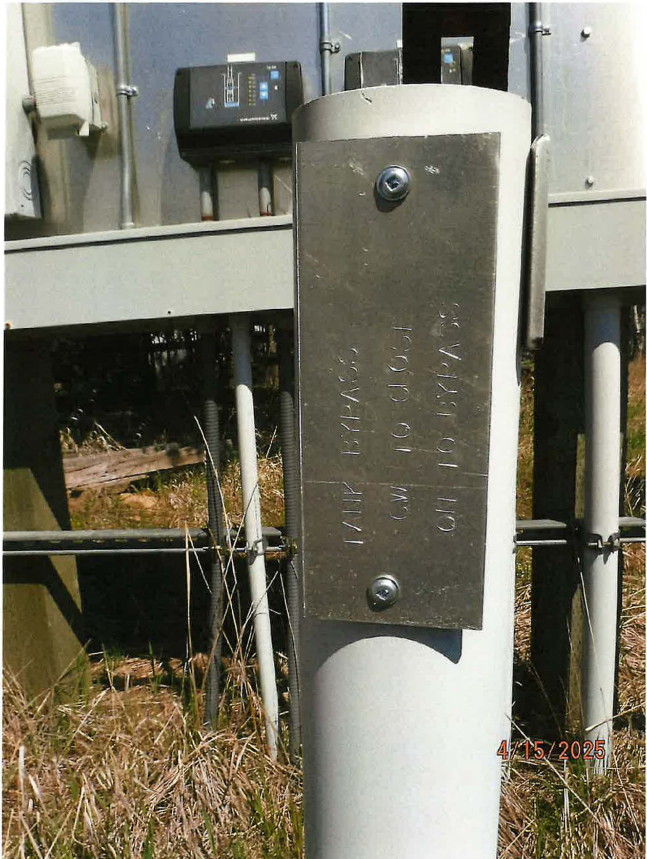
TANK BYPASS VALVE
