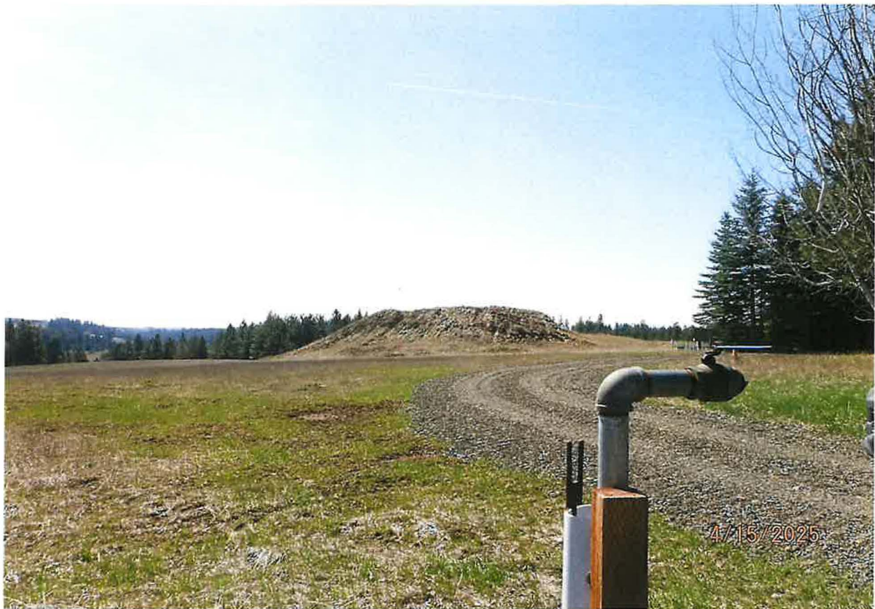
FIRE PROTECTION POU – 2-INCH FIRE TENDER FILL POINT
