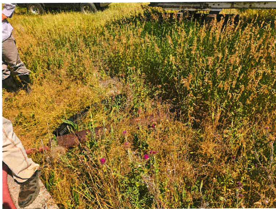
Figure 8 Cistern inlet lines.
