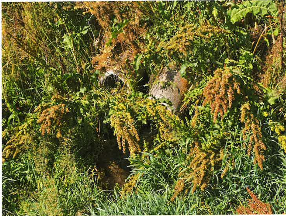
Figure 9 Outlet for the right head gate that feeds into the active stream channel. On the right side is the active release point.
