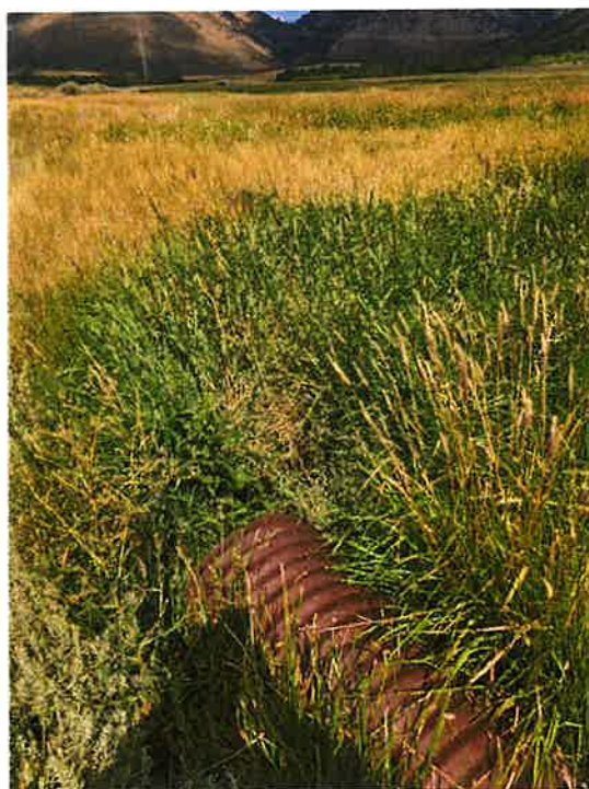
Figure 4 Culvert at the midpoint of the POU.
