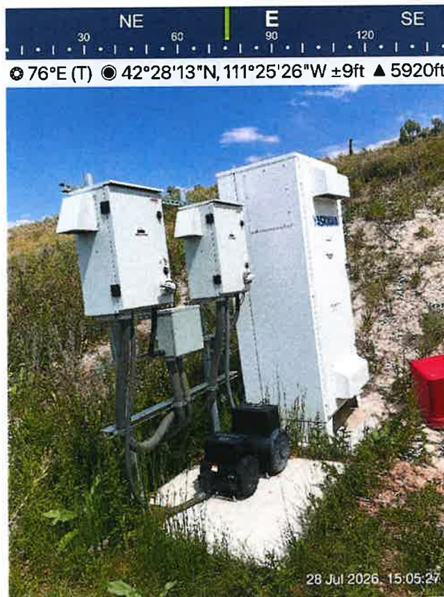
Figure B: Electrical system that supplies the pump.
