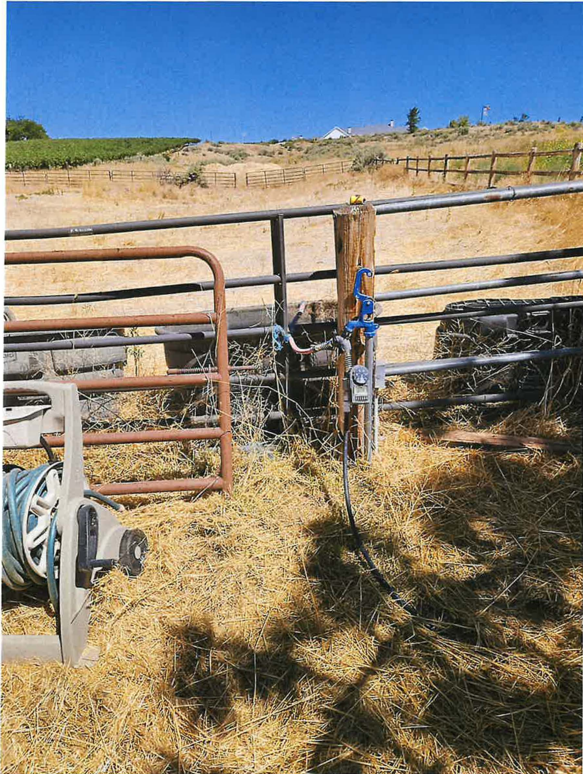
Photo of stockwater diversion works from 8/11/2025 email correspondence: “RE: Additional Information Need to Proceed with Water Right License - Water Right No. 63-33955”
