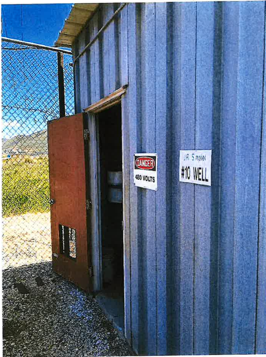
Well #10 outside building
